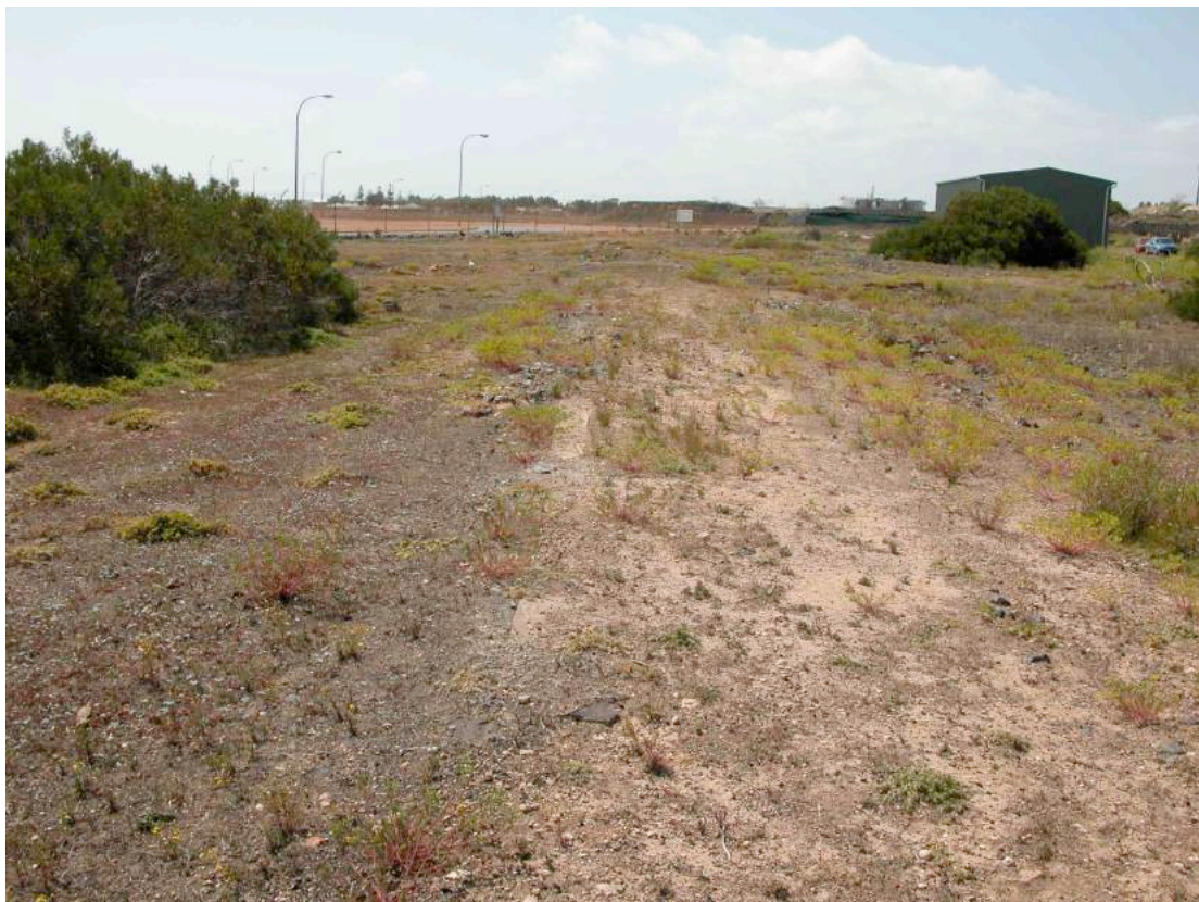
Fig 42 One of the 200m-long coal gantry track foundations, looking north (see Fig. 17, p. 23)
