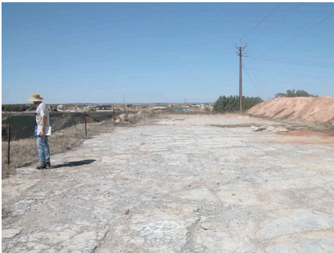
Fig 34 The paved area on the upper level near the north end of the retaining wall is the charge floor where the blast furnaces standing on the lower level (at left) were fed (see Fig 13, p. 21)
