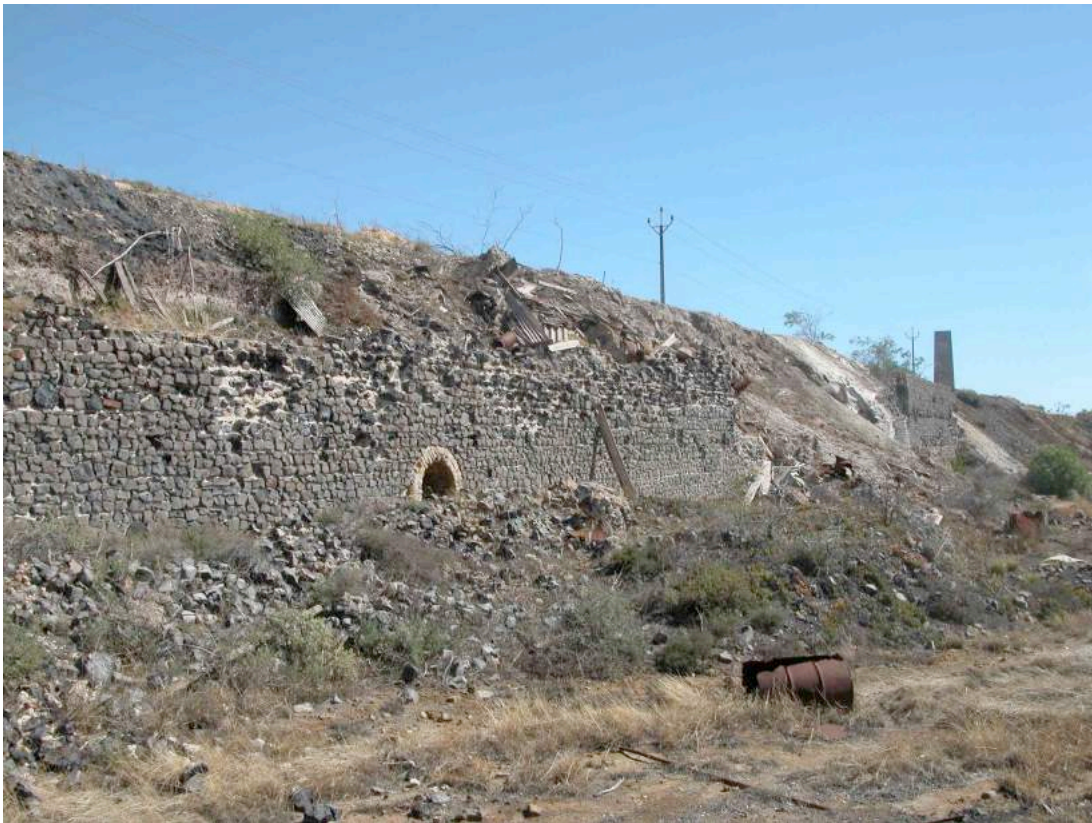
Fig 29 The retaining wall is a dominant element of the site, over six metres high in places, some of its length formed of two walls with internal flues from the furnaces between them
