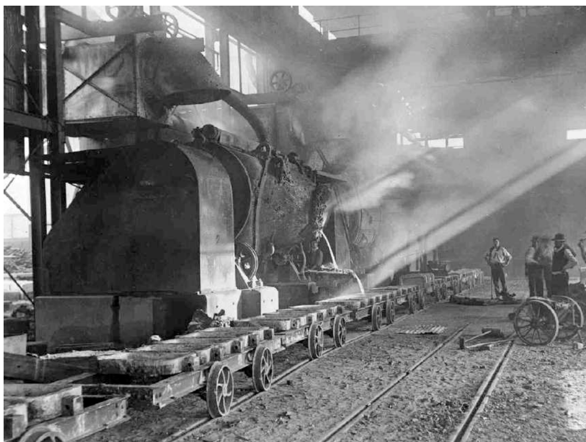
Fig 21 Pouring copper ingots from a converter (PIRSA N010755a)
