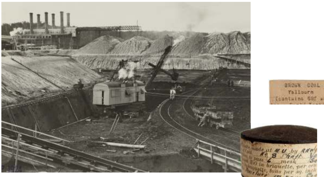
Figure 1: Bucyrus Type 175B 3½ cubic yard capacity steam shovel engaged in early coal winning with Yallourn A Power Station in background, 1925; Yallourn lignite sample (E 7604); Experimental Briquette, circa 1921 (HT 56098) Sources: SECV Image Collection; Mineralogy Collection, History & Technology Collections, Museums Victoria.
