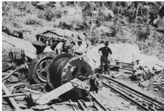
THE CABLE DRUMS, BLOWN 50 FT. FROM THEIR FOUNDATIONS.
