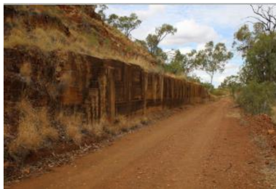
Hightville ore transfer stage, Ballara Heritage Trail, where ore was loaded onto railway trucks
