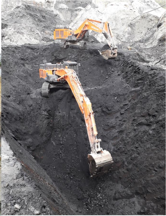
Structurally Thickened coal
