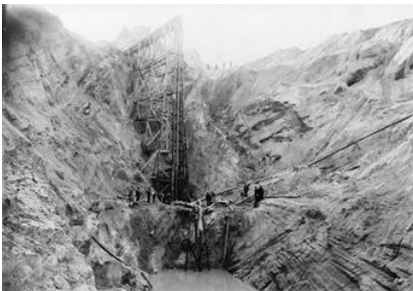
Figure 16. Hydraulic elevator, St Bathans, ca. 1890s. This elevator was used to pump gravels from the pit to a higher level for processing and extraction of the gold. It operated until 1934.
