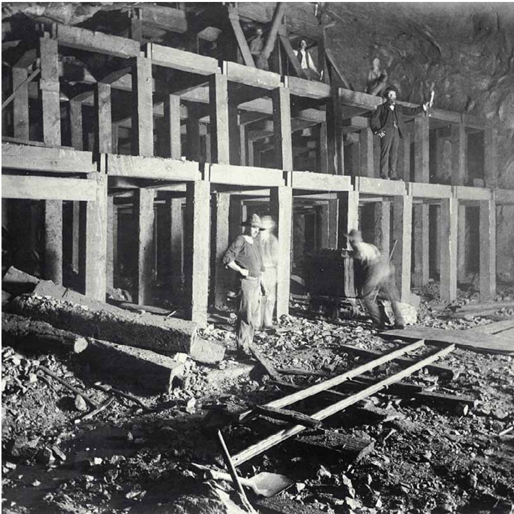
Set-square timbering, BHP Mine, Broken Hill, 1890.
