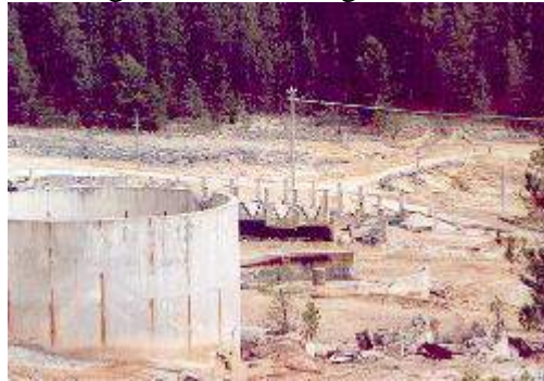
Remains of the flotation plant
