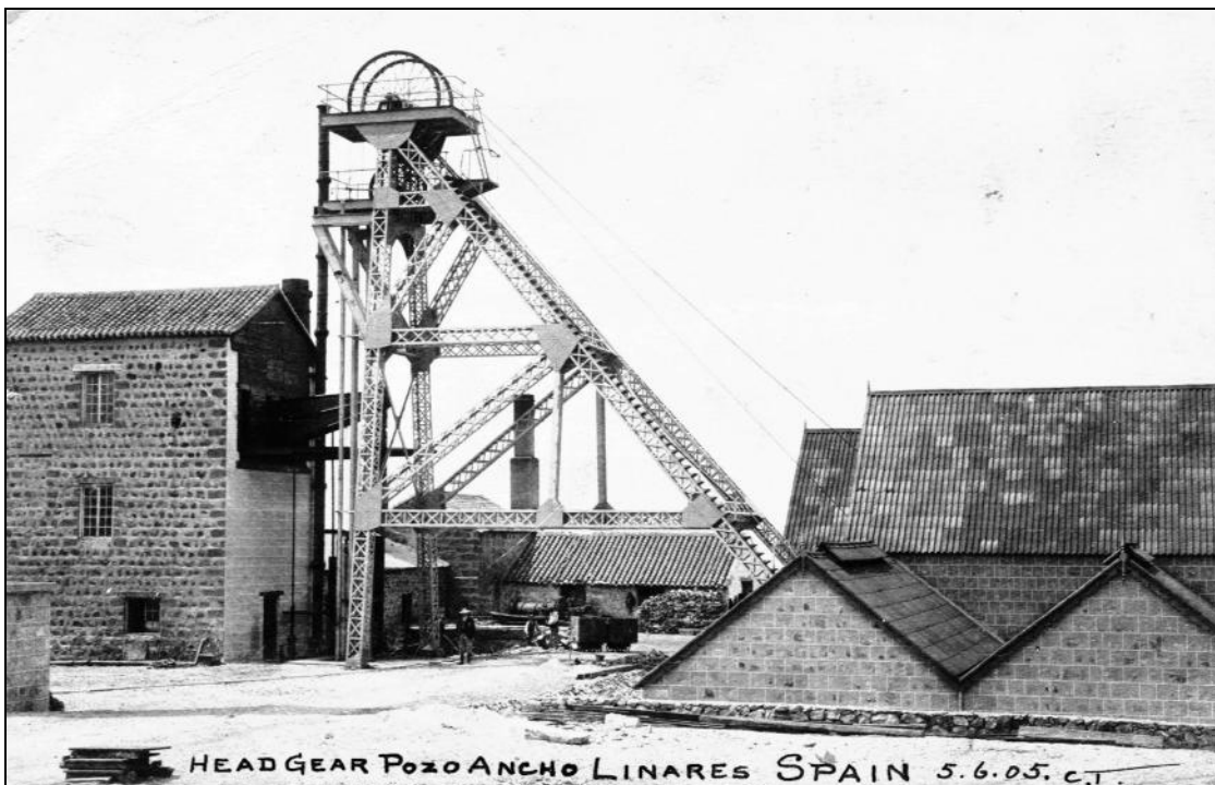
Figure 7: Piell's shaft, Pozo Ancho mine, Linares Lead Mining Company Limited: The Cornish type pumping engine house together the new headframe and winding engine house installed in 1904.
