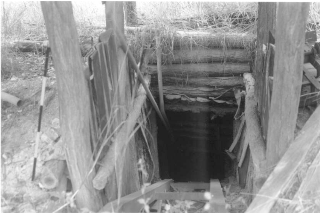
Figure 8: An example of an underlie shaft sunk in the 1980s on the Waitemata mine site
