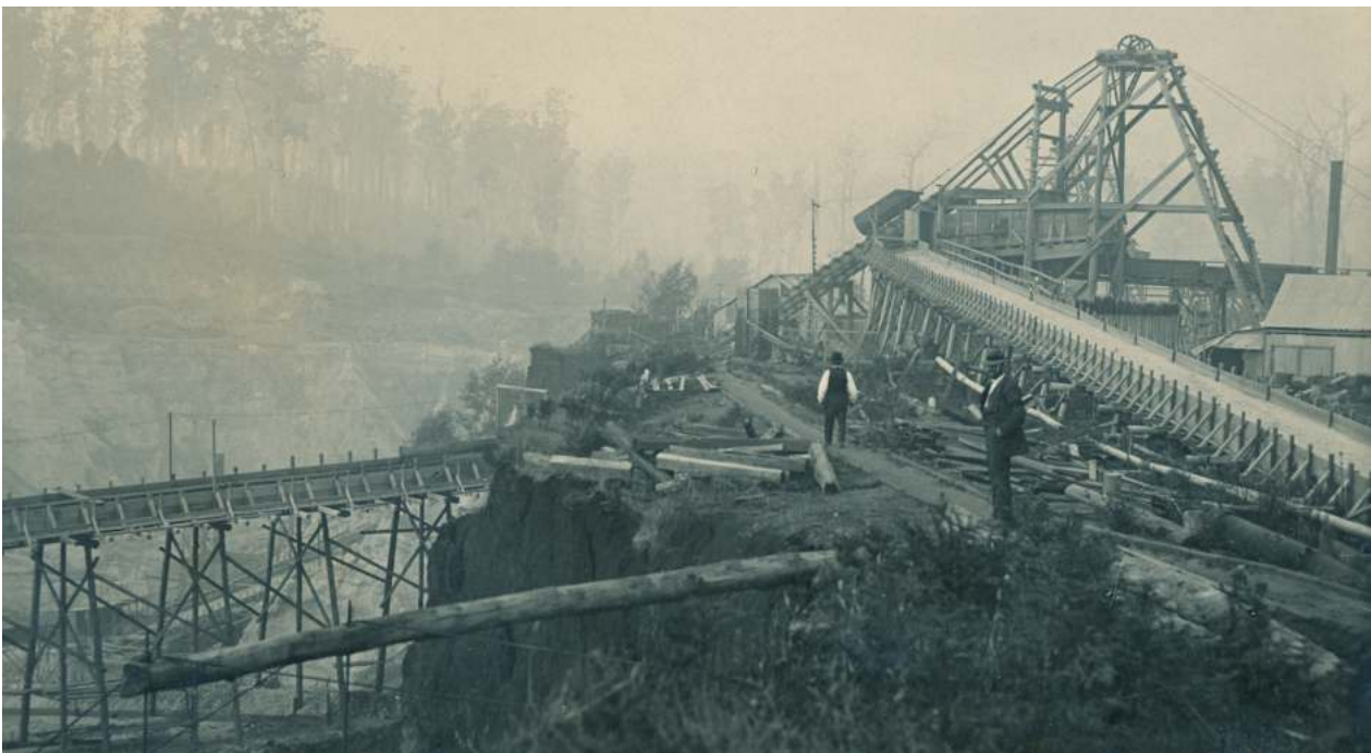
Figure 6: Headframe for steam winding engine on the No. 3 Incline. Figure in the foreground possibly mine manager Mitchell.
