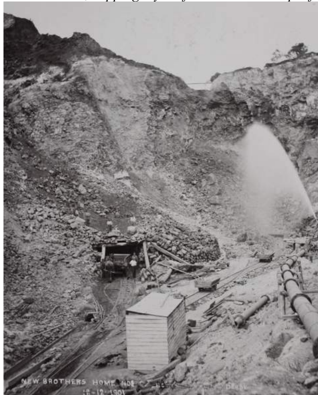
Figure 5: Overburden removal from the NBH1 Co. lease by a combination of hydraulic sluicing and trucking of large basalt blocks, capping layer of Briseis Hill in top left corner.
