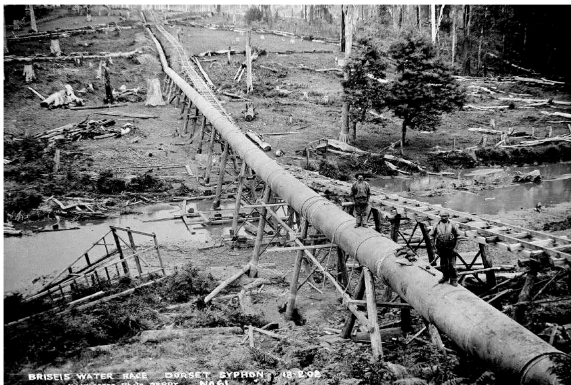
Figure 7: Dorset Syphon with construction tramway.
