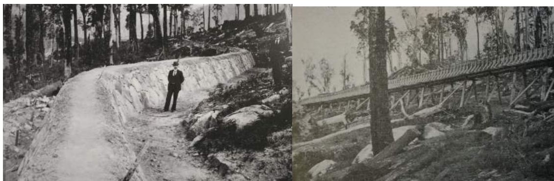
Figure 8: Stone-faced bundwall & flumed sections of the Ringarooma Race.
