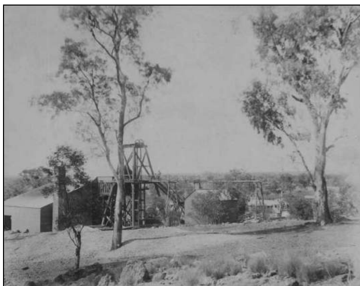
Figure 2: View of the Girilamborne copper mine with new poppet head, looking northeast ca. 1896. Houses in the mine town can be seen in the far background.
