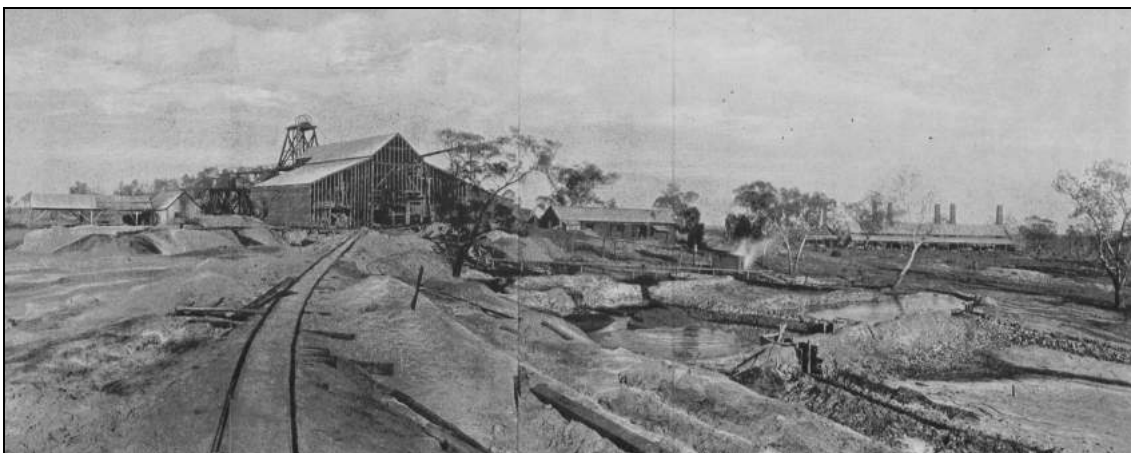
Figure 6: View looking southwest of the Girilambone copper mine and works at the time of J.E. Carne's inspection in 1998. Concentration plant at centre in front of main shaft head frame and smelting plant far right
