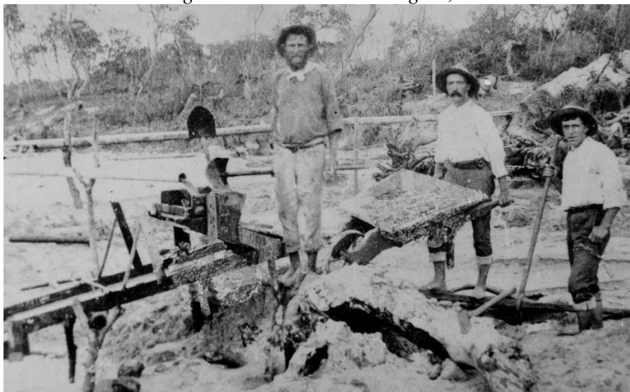
Figure 2: Beach miners using a sluice box to recover gold, Ballina ca. 1890.
