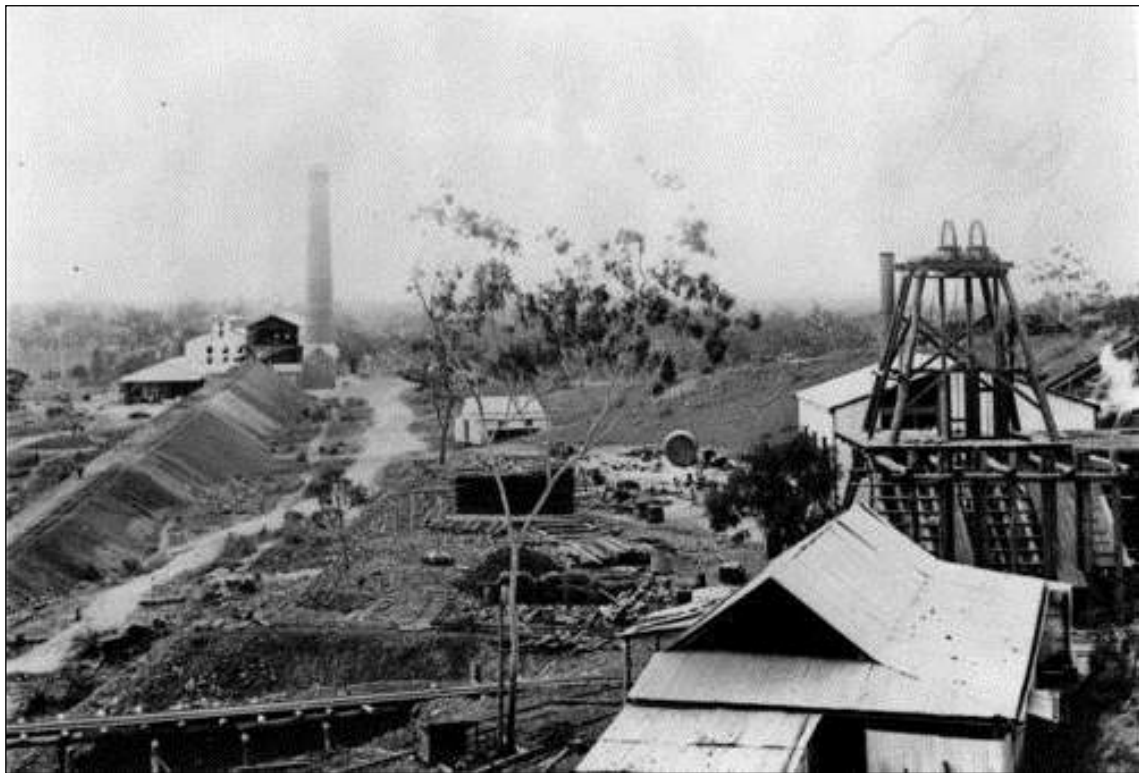
Figure 2: The mine in 1901. The 'Tunnel' is to the right of the headframe, and the trestle in the foreground leads to the main ore bins on the left.
