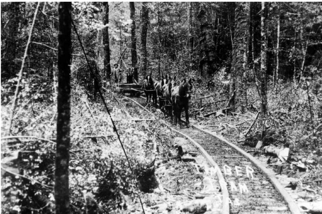
Figure 3: The V.D.L. Co.'s timber tramway operating in the Nine Mile Forest south of Burnie. This horse-drawn tram working on wooden rails shows the technology used on the Mount Bischoff Tramway.
