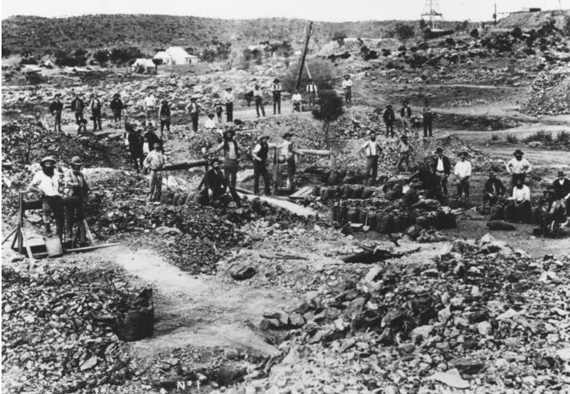
Figure 2: Thackaringa mines 1883, showing mining methods and settlement in background.
