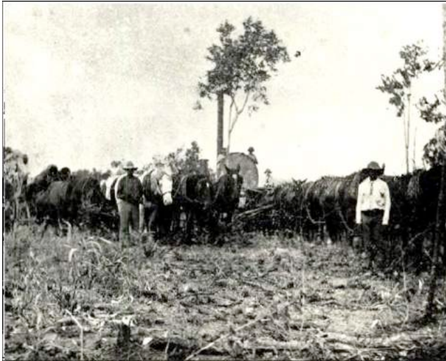
Figure 5: Figure 5: Carting Sluicing Pipes from Lara to Palmerville.
