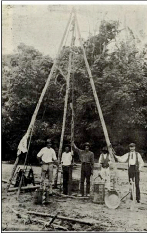
Figure 6: Boring for tin on the Romeo Company and Carson Dredging Claims.
