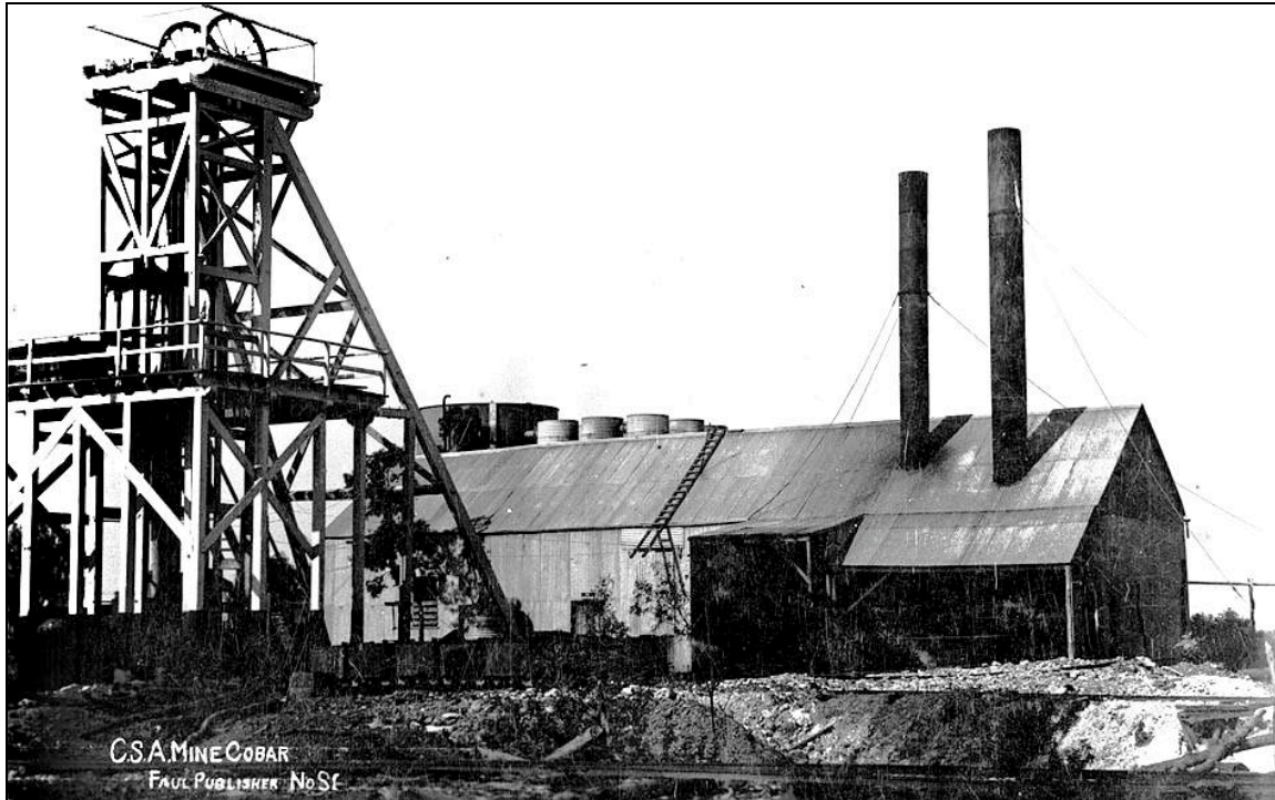
Figure 5: The C.S.A. main shaft headframe and engine house ca 1918, view looking northeast.
