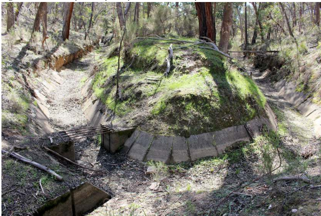
Figure 5: Junction of Poverty Gully Channel with Fryer’s Channel.
