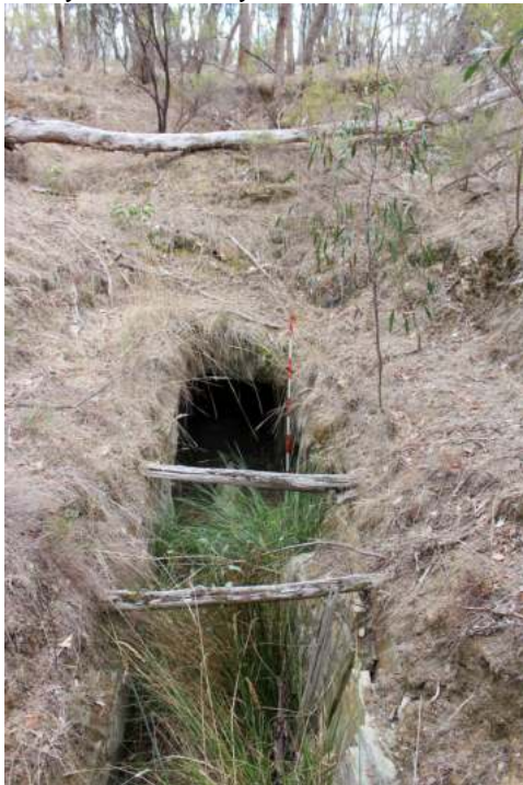
Figure 3: Southern entry to Devil’s Gully Tunnel, Fryerstown.
