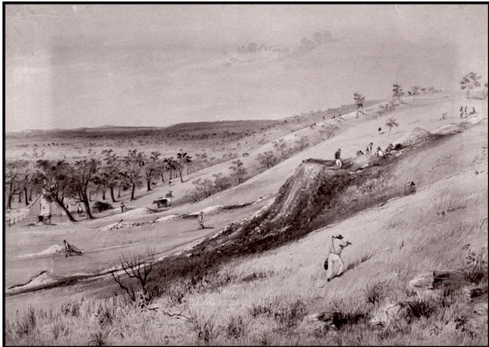
Figure 3: S.T. Gill Glen Osmond Mine 1845 showing Victoria shaft.
