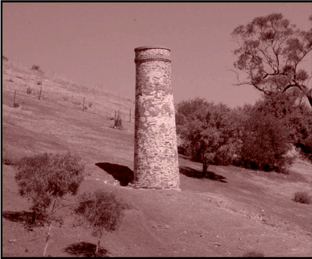
Figure 8: Glen Osmond smelter chimney.
