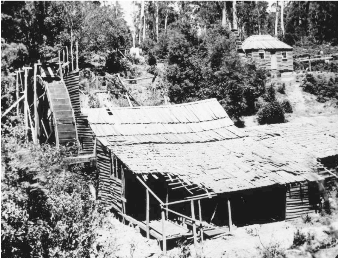
Figure 3: Battery on the Enterprise Co. claim driven by an iron-framed overshot waterwheel, photograph probably dating from the 1890s when disused.
