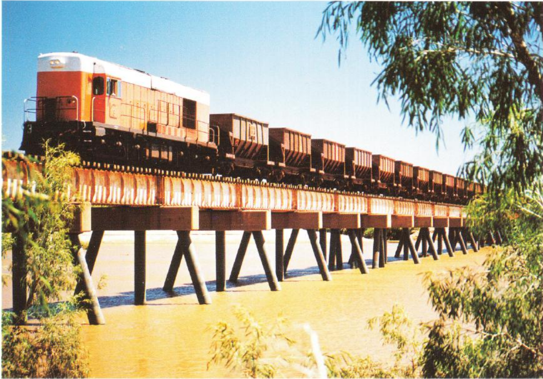
Figure 1: De Grey River Bridge.
