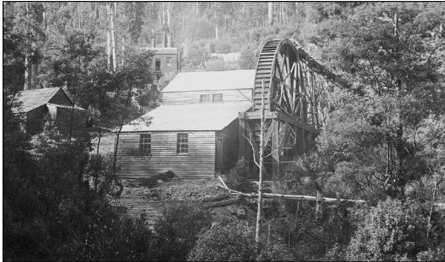
Figure 3: Mercury battery driven by a pitchback water wheel incorporating an iron shroud and buckets.
