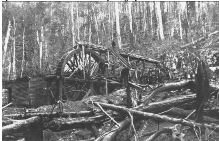
Figure 6: Official opening ceremony of the first Long Struggle battery driven by an overshot waterwheel of largely timber construction, 1922 - 23.
