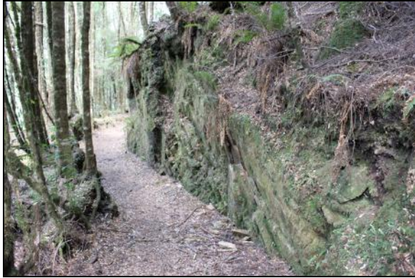
Figure 5: Water race formed in a rock cutting adjacent to Philosopher Falls (WR 2228W) – part of short section restored for use as a walking trail.
