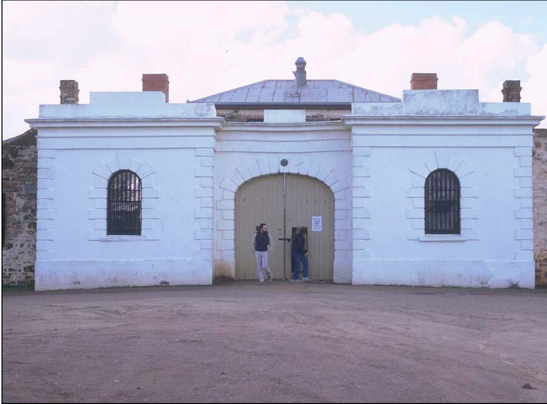
Figure 6: Redruth Gaol, constructed 1856
