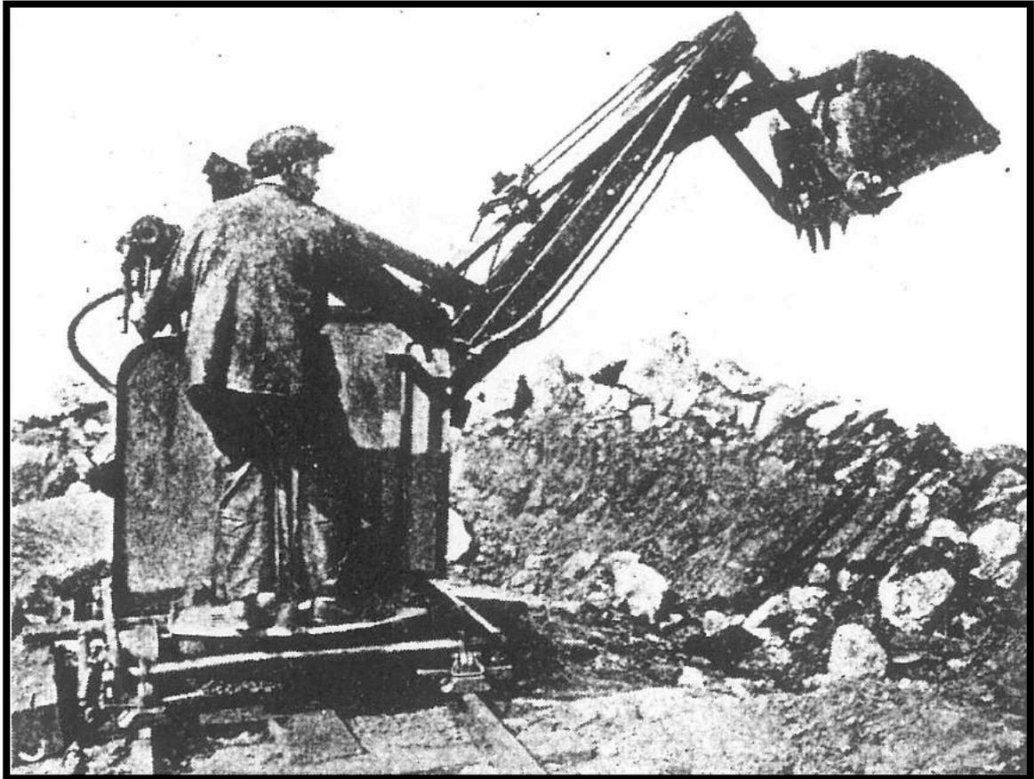
Source: Mechanical loading in tunnels and mines, *Chemical Engineering and Mining Review*, September 5, 1927, p. 453.
