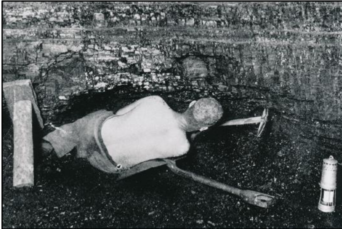
Figure 5: Undercutting by hand in one of the Bulli district collieries, ca. 1949.
