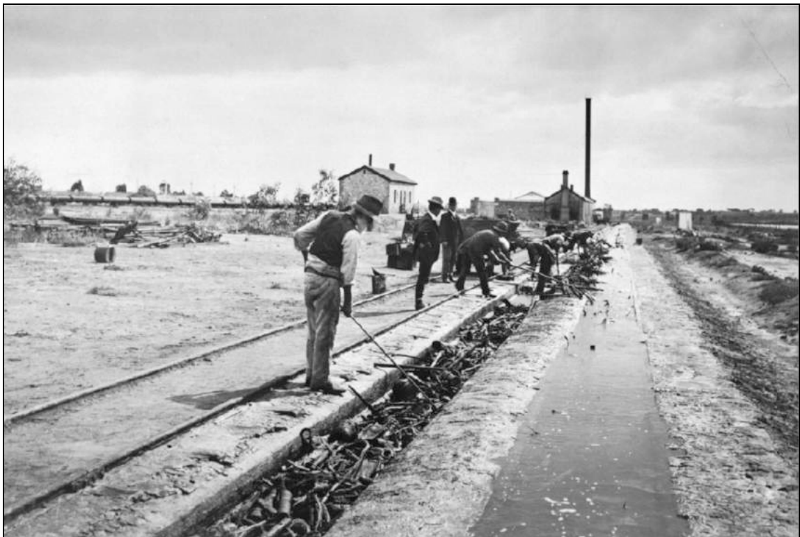
Figure 6: Cleaning out scrap iron from a precipitating canal.
