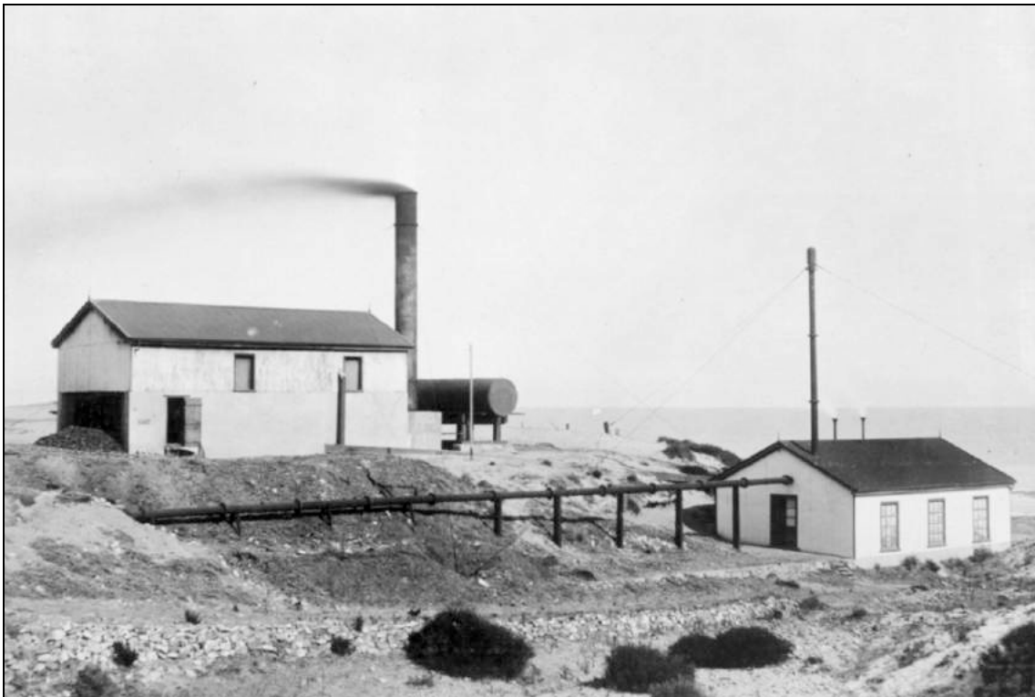
Figure 1: The Pumping Station at Rossiter's Point on Moonta Bay.
