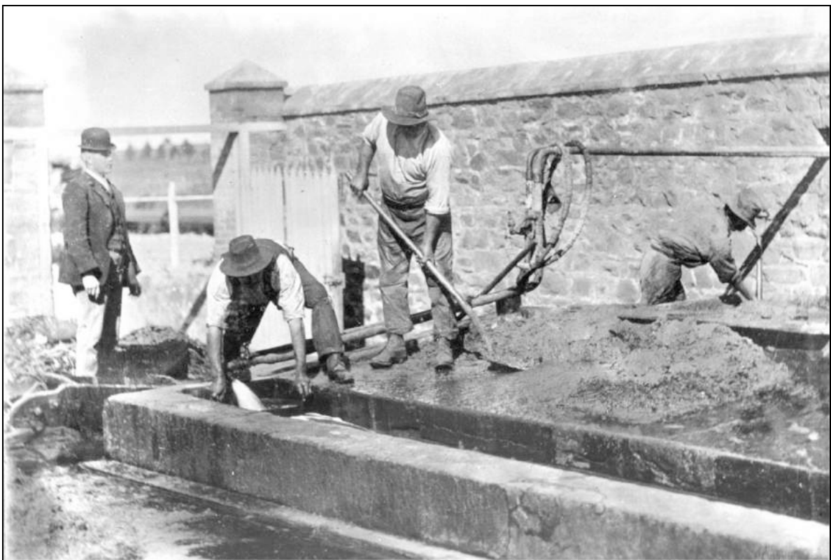
Figure 3: Removing precipitate from the canals at the Wash and Dry House.
