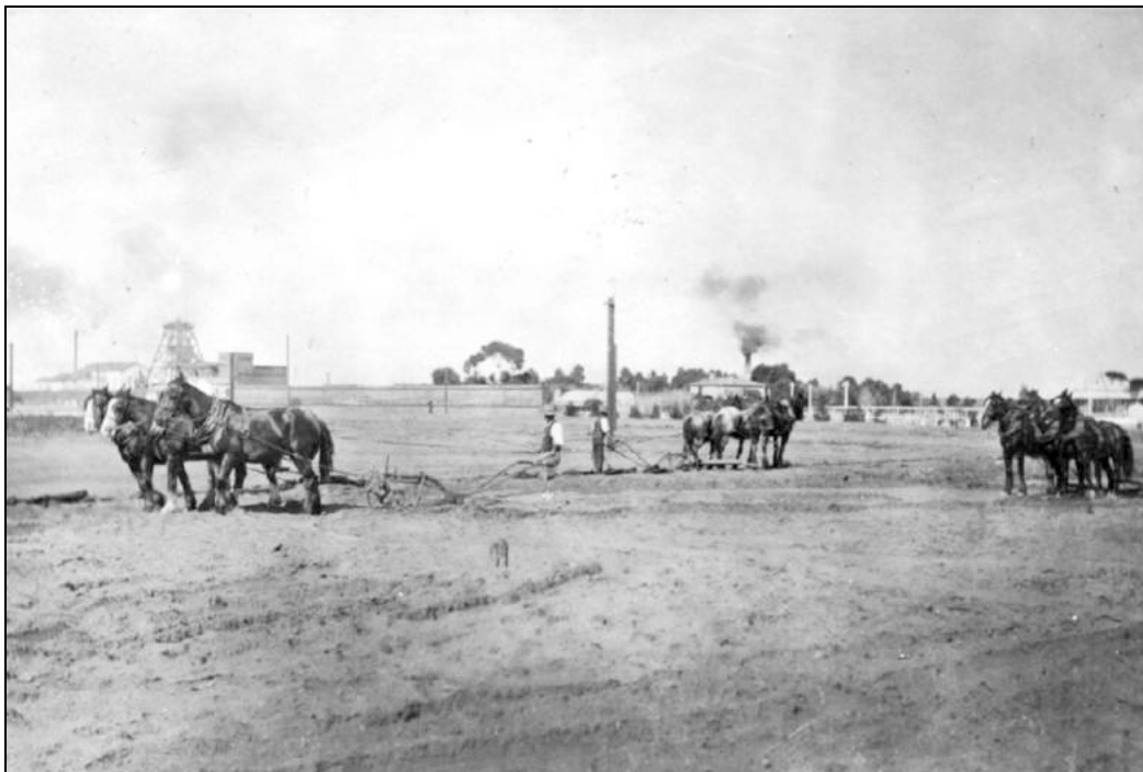
Figure 5: Ploughing the slimes to encourage oxidation.
