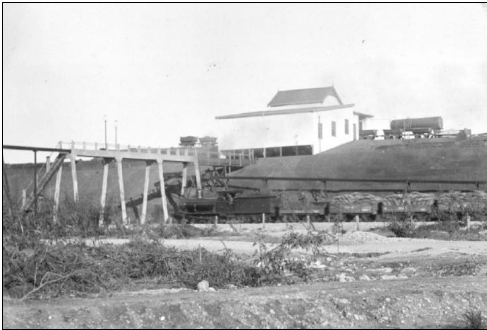
Figure 4: The Slimes Treatment Plant situated on Ryan's Heap.
