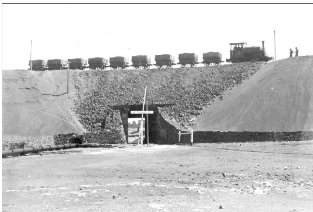
Figure 7: The Tramway Tunnel through Ryan's Skimps Heap.
