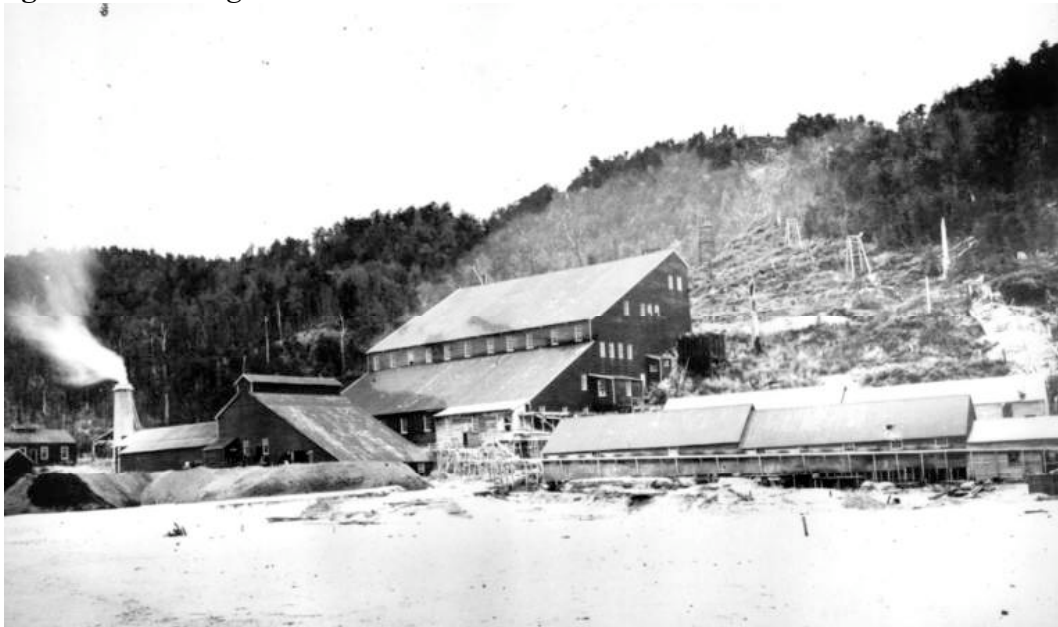
Figure 2: The Progress Treatment Plant
