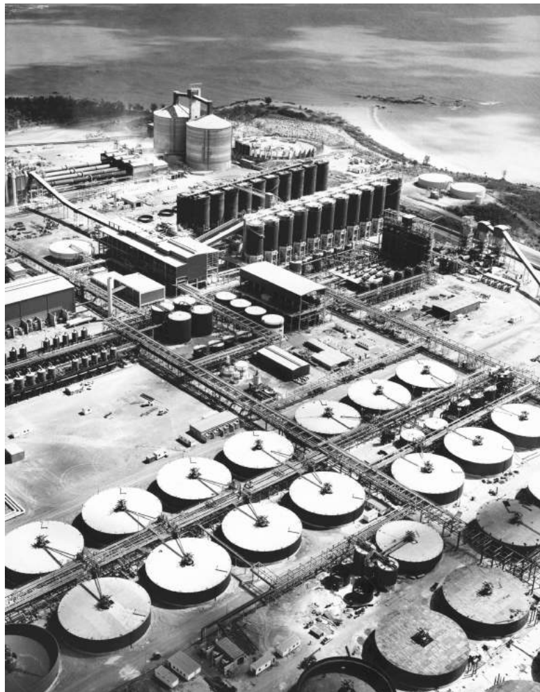
Figure 1: Nabalco Bauxite and Alumina Plant, Gove, Arnhem Land, General view of alumina plant 1972
