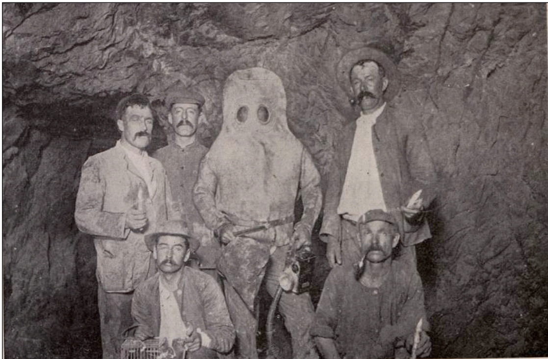
Figure 2: 'Flashlight photograph showing Smoke Jacket and Air Hose, and illustrating method of sampling air in connection with experimental blasts at Kalgurli Gold Mines Limited, Kalgoorlie, and cage used for tests on animals'.
