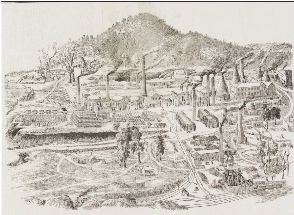
Fig. 1: Lithgow Valley Colliery Co's Brick and Pipe Works with Lithgow Valley Colliery in foreground.
