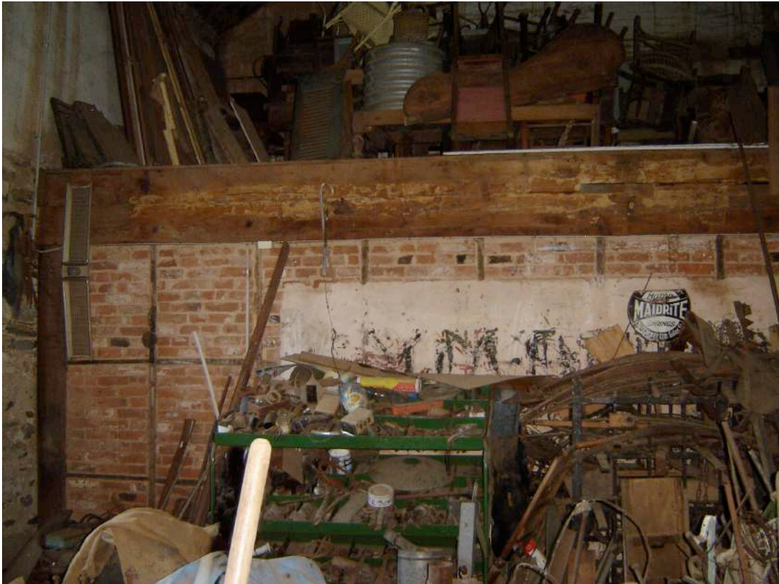
Figure 7: The nogging wall bounding the insertion from the southern lean-to of two bedrooms into the main chamber under the foreshortened mezzanine floor.
