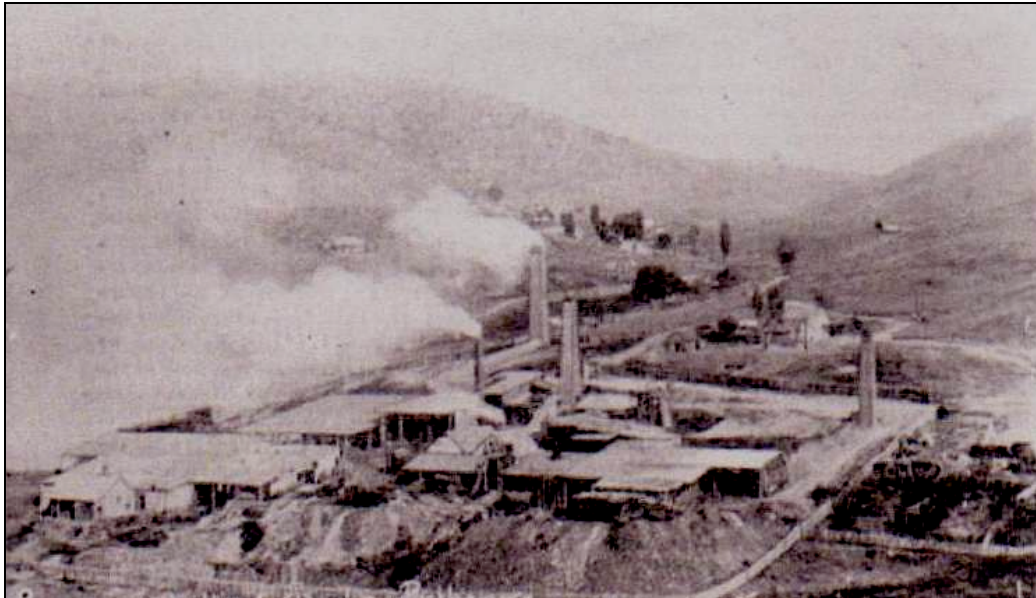
Figure 6: Wallace Bethanga Chlorination Works, circa 1897.
