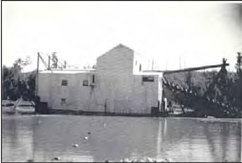
The Snowy River Gold Dredging Ltd dredge at work. The dredge is digging ahead to the right, and the pond is being filled in by the debris behind the dredge at left. Note the sluice box discharge (at the extreme left of the picture) which resulted in the restoration of the dredged ground.
