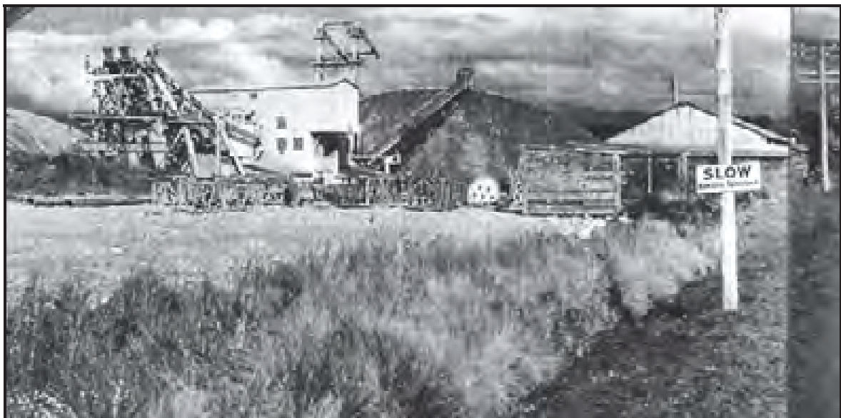
Kaniere dredge operating on Tucker Flat in the vicinity of the Kaniere township. Work ceased in 1953. The dredge was then dismantled and rebuilt near Kumara where it worked down the lower Greenstone into Teremakau River from 1956-1981.
