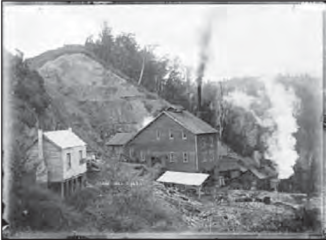
Progress or "B" shaft. The winding engine was housed in the lean-to at left, blacksmiths shop to right and preparation area for mine timber in the foreground.
