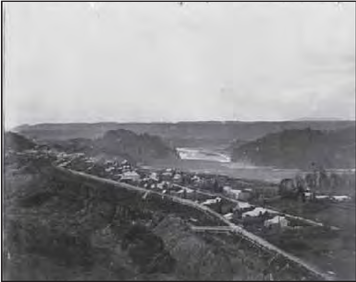
View of Dillmanstown from the southwest with Dunedin Flat workings in the foreground. Kumara Government water-race crosses middle of photo.
