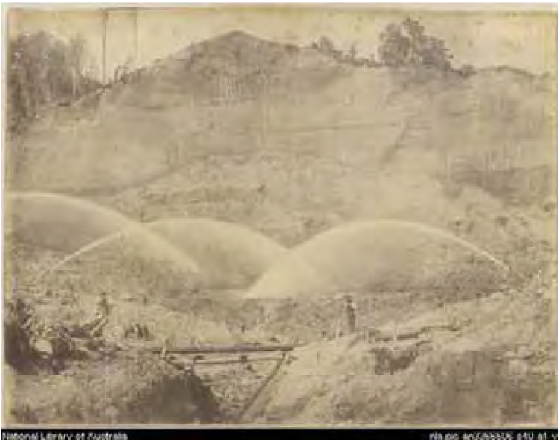
Humphrey's Gully sluicing claim in 1885. One of the largest sluicing claims on the coast it was serviced by a 12 mile long water-race.
