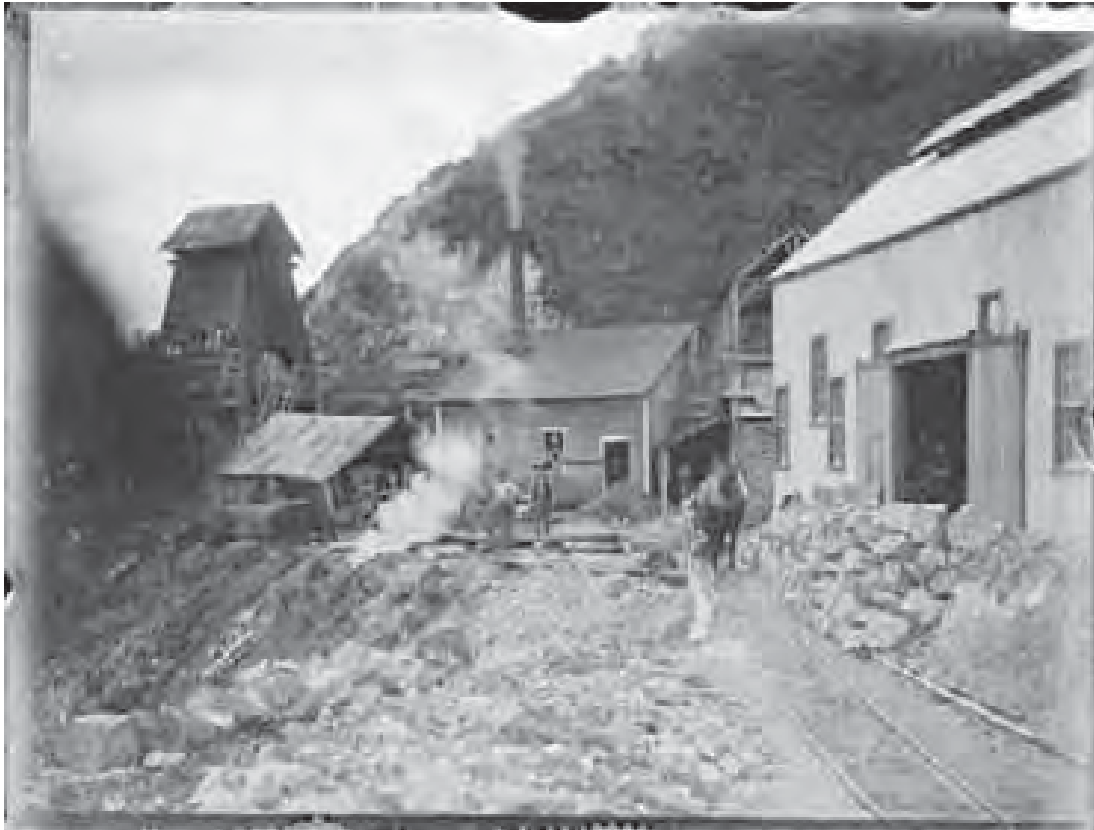
Globe or “A” shaft buildings. The shaft, sunk by the Globe Mining Company, was directly below the head frame at left. Engine house for the steam-powered winder is in the centre of photograph.
