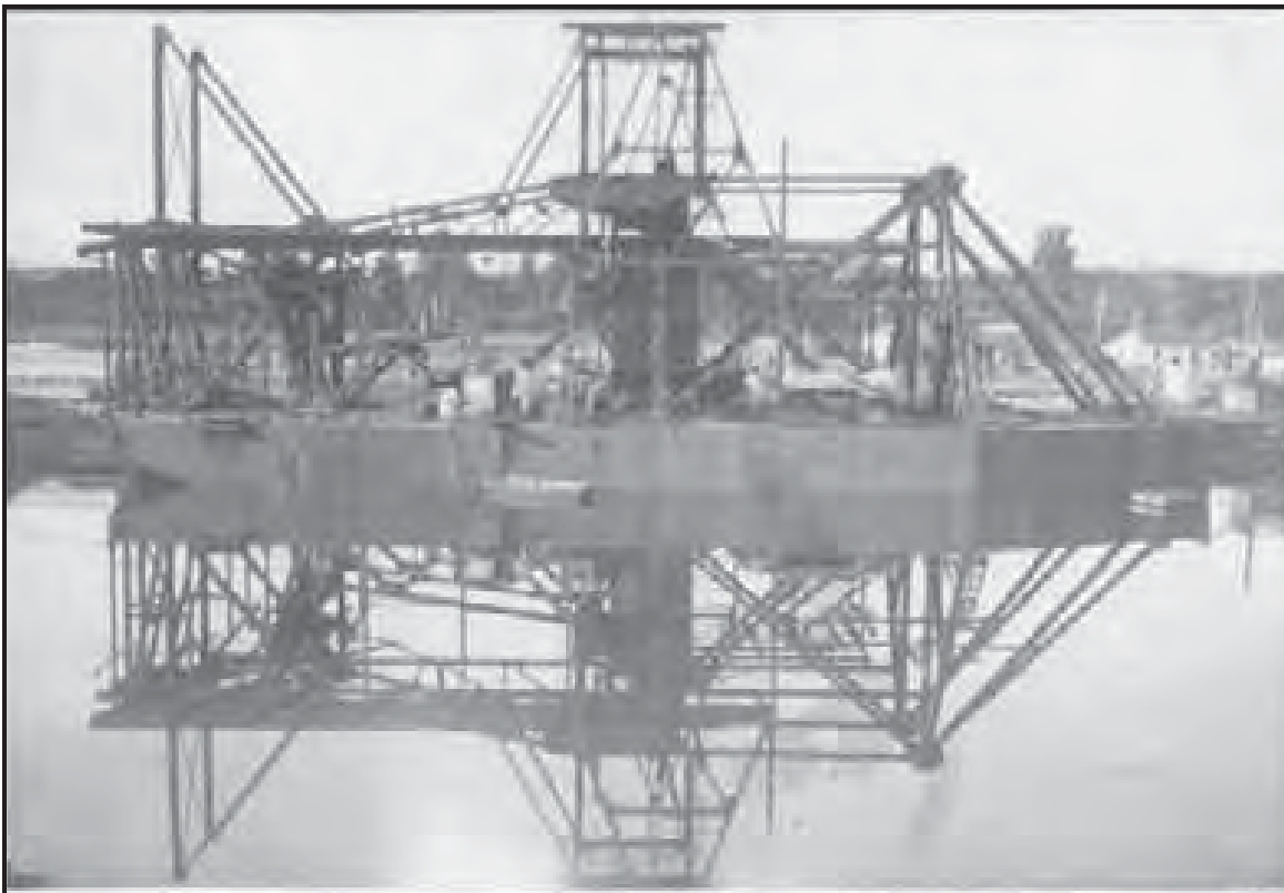
View of the pontoon and superstructure of the "Big Grey" after the sideways launching on 23 April 1938. Steelwork was fabricated by Andersons Ltd who were also responsible for the construction of the Snowy River Gold Dredge. Ikatamua township in the background.
