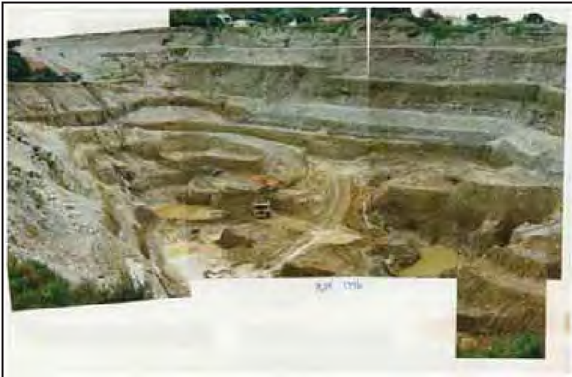
Birchfield Ross Mining Ltd., openpit, 1996, on the southern edge of Ross. Total depth 85m. The excavator is an 80 tonne machine. Five "bottoms" with very coarse gravels can be seen in the pit wall. (R.J. Cotton photograph).
