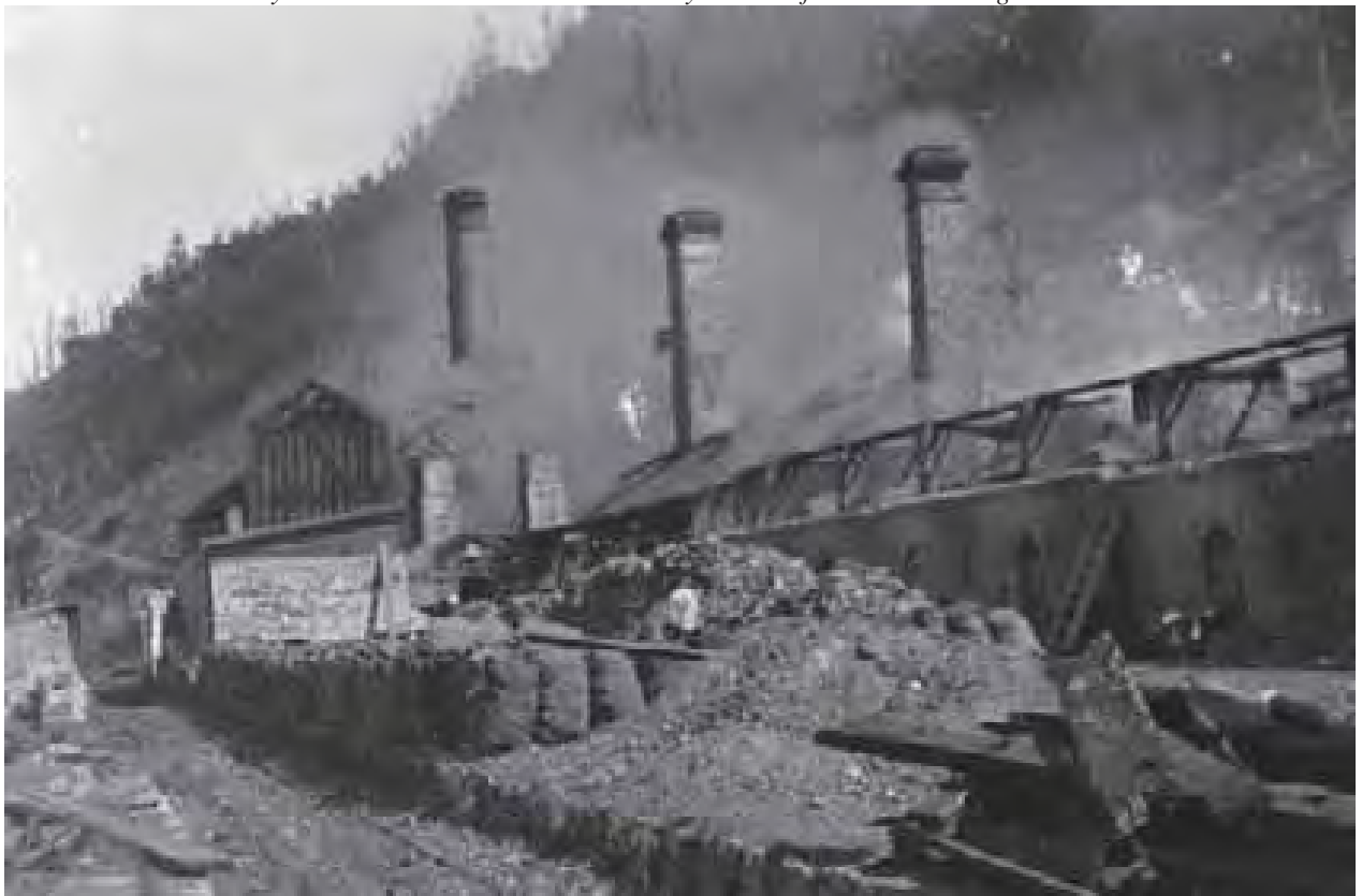
Plate 2 Beehive coke ovens adjacent to the Brunner Mine. After closure in the 1930s the ovens were abandoned and eventually overgrown with native bush. Under the care of the Historic Places Trust the ovens have been cleared, stabilised and protected and now form part of an industrial archaeology complex.
