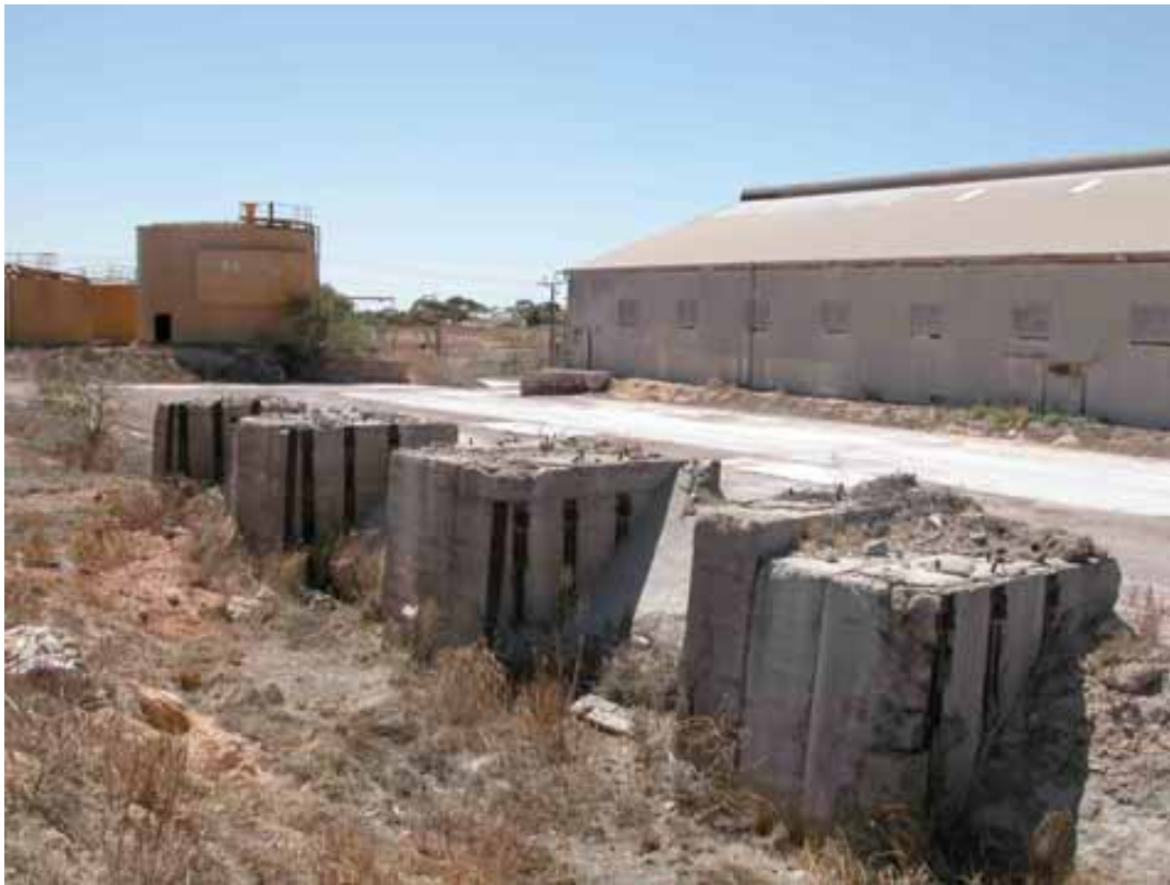
Fig 33 The foundations of the McMurtry sintering pots stand on the upper level (see Fig 19, p. 24)
