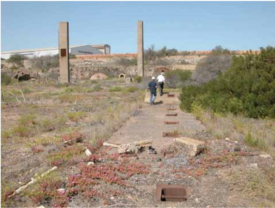
Fig 41 The underground coal conveyor runs from the coal gantry to the pulverising plant
