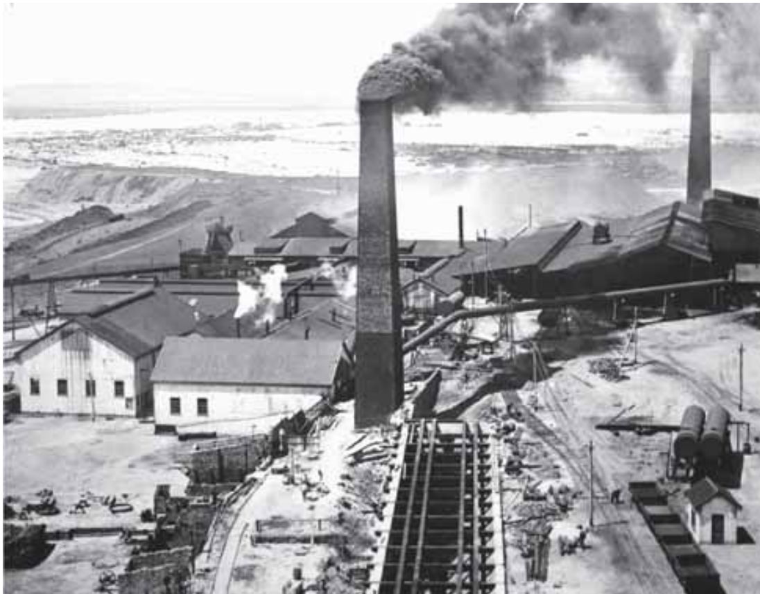
Fig 18 General view of smelters from Hughes Stack in later years: powerhouse and electrolytic refinery at left, converter shed at rear, blast furnaces and sintering pots in large shed at right (PIRSA 038613a)
