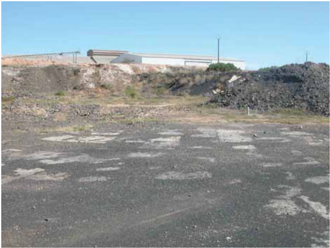
Fig 43 The extensive slag-paved floor of the coke depot
