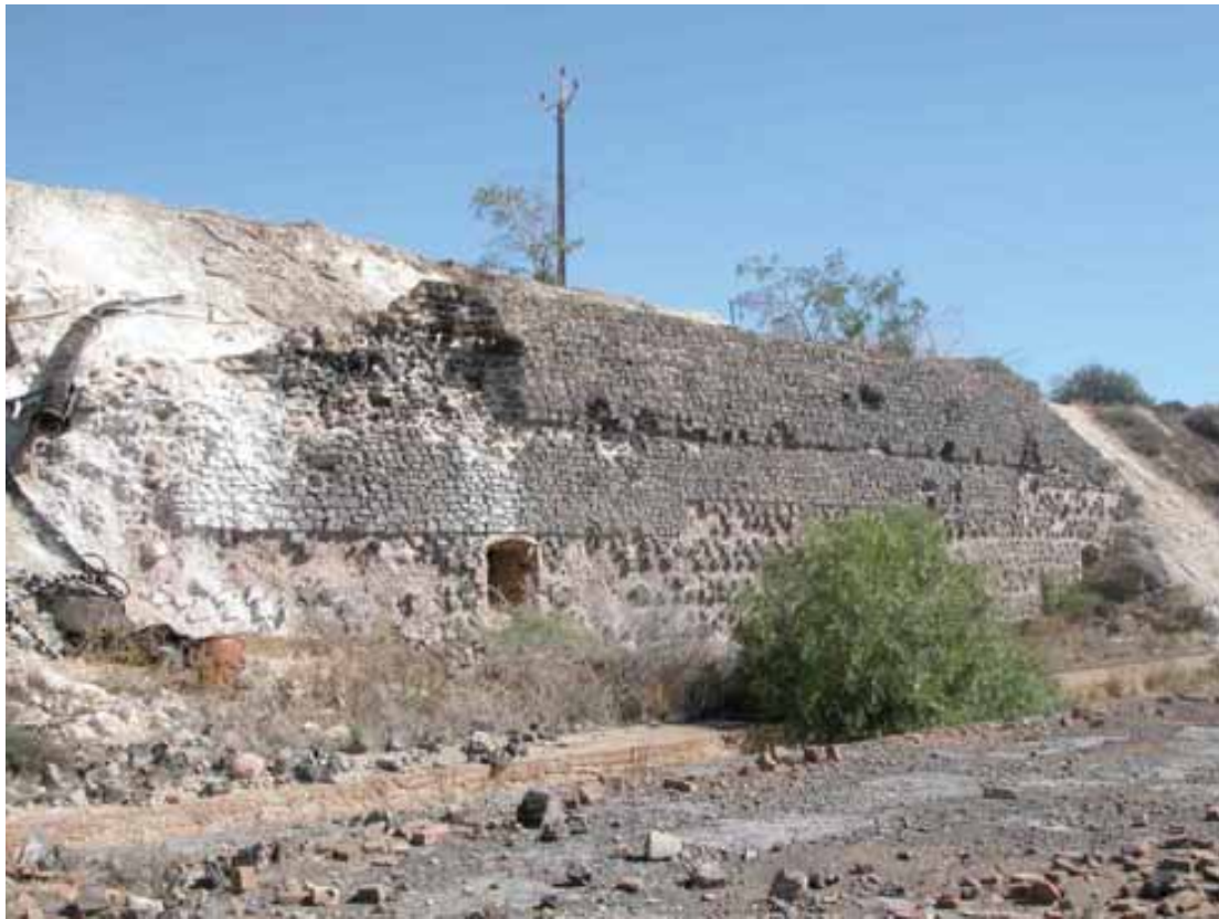
Fig 35 The foundations of the blast furnaces stand below the highest section of retaining wall
