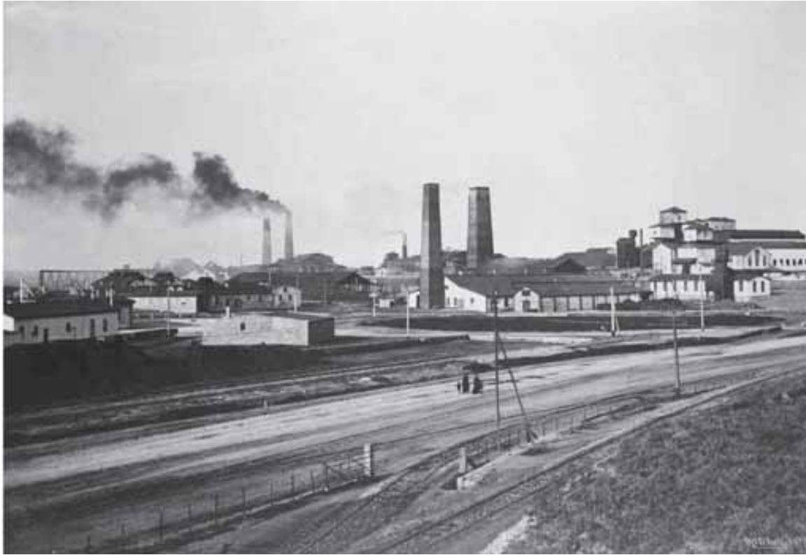
Fig 10 General view of smelters c.1910, sulphuric acid plant on right (PIRSA N007158a)
