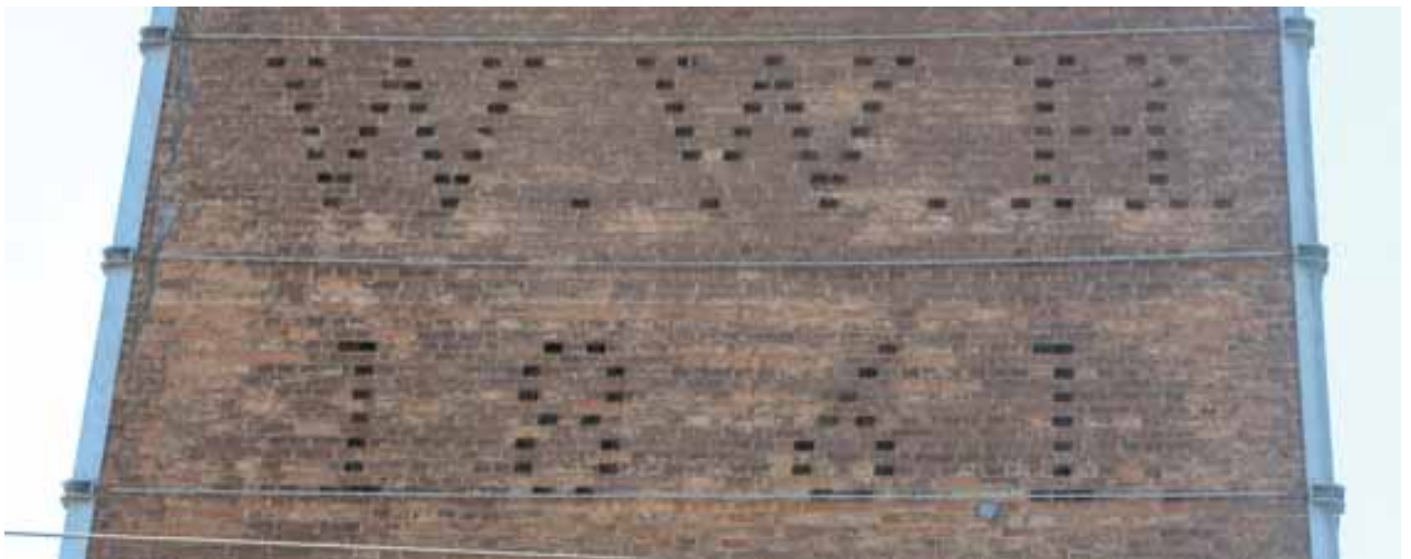
Fig 28 Walter Watson Hughes' initials and the year of construction are picked out in the brickwork on the east face of the stack
