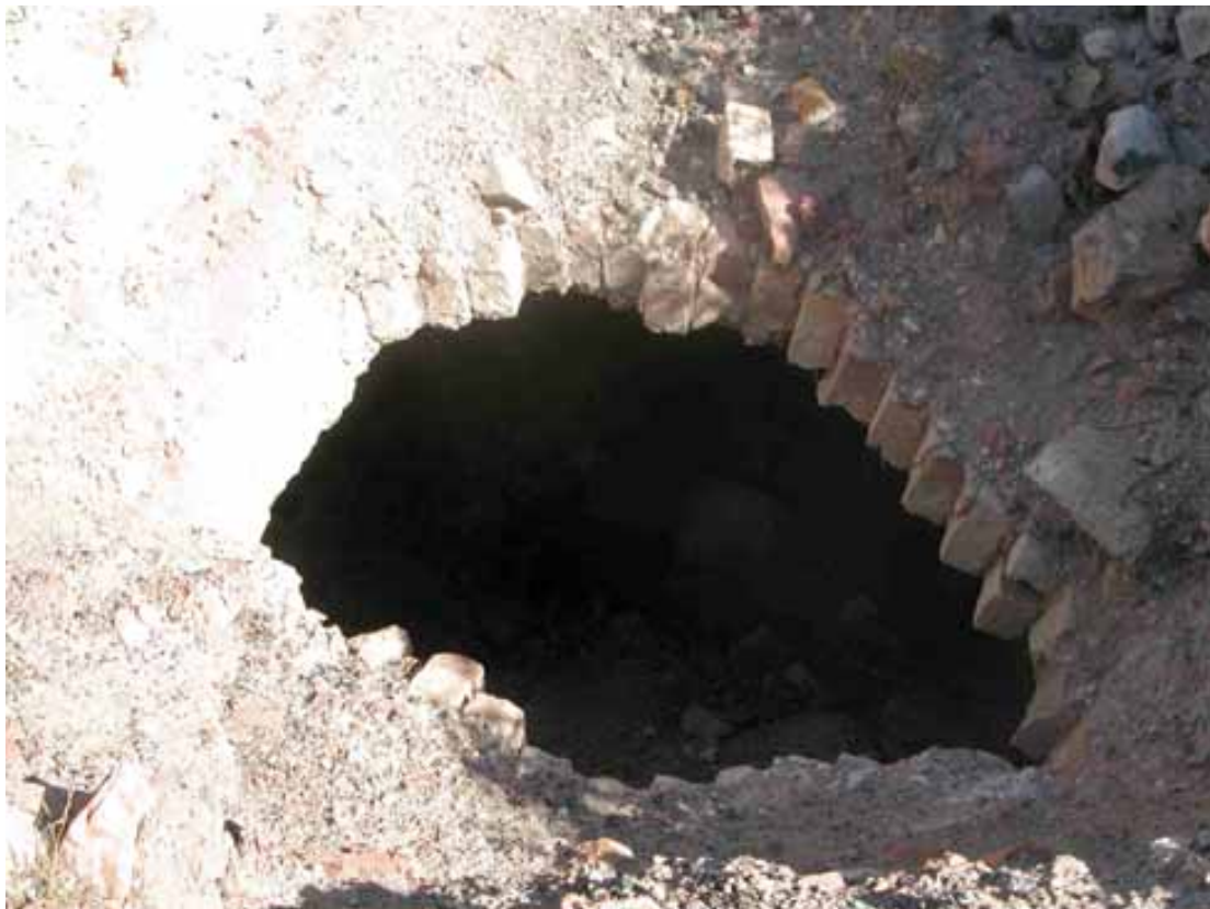
Fig 32 The furnace area west of Hughes Stack has extensive underground flues
