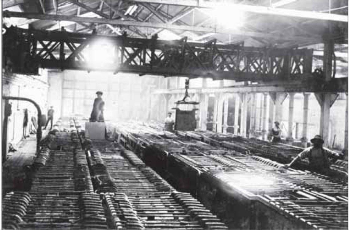
Fig 16 The electrolytic refinery, showing rows of anodes in the tanks (PIRSA N020505a)
