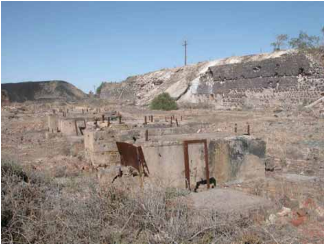
Fig 37 The foundations of the converter plant on the lower level (see Fig 21, p. 25)
