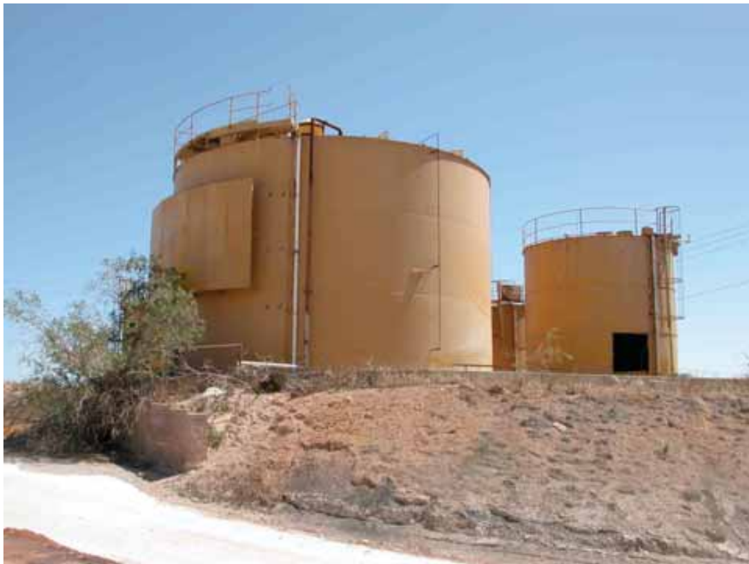
Fig 48 Most of the fertiliser factory's infrastructure dates from recent decades
