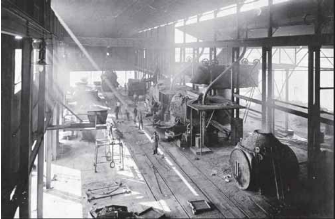
Fig 20 Looking down into the converter shed (PIRSA 034035a)
