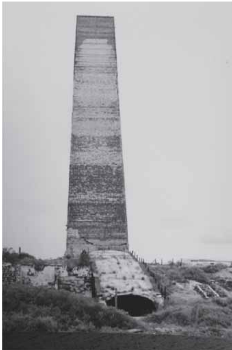
Fig 24 Hughes Stack, looking east, April 1975. The section of flue visible in the foreground was demolished before 1985 (National Trust file 1834)
