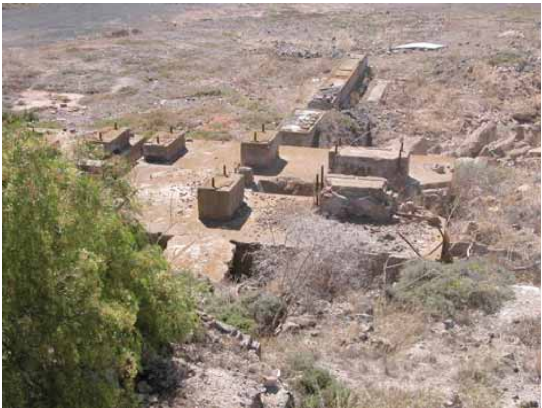
Fig 38 Power house engine and generator foundations, looking west (see Fig 14, p. 22)
