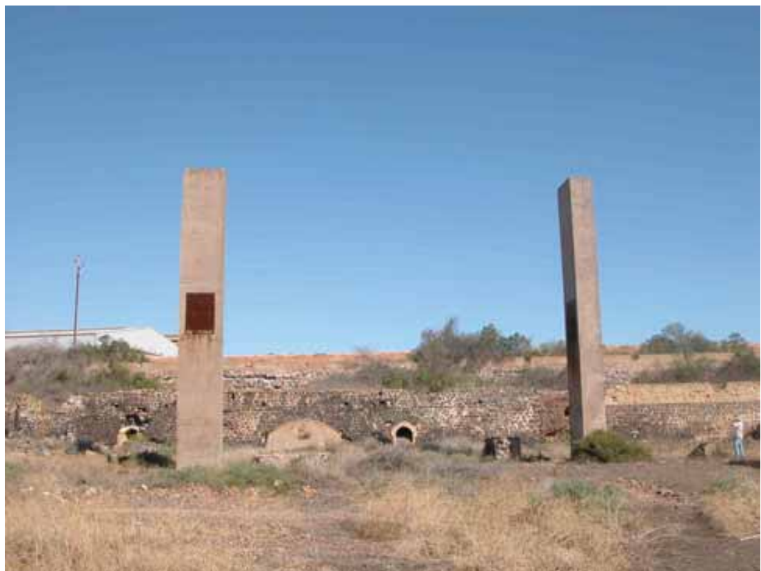
Fig 40 Air lift shafts from the coal pulverising plant are among the most conspicuous relics on site
