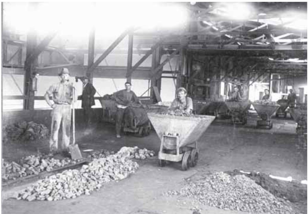
Fig 13 The charge floor, ore and coke being loaded into the blast furnaces (PIRSA N020511a)
