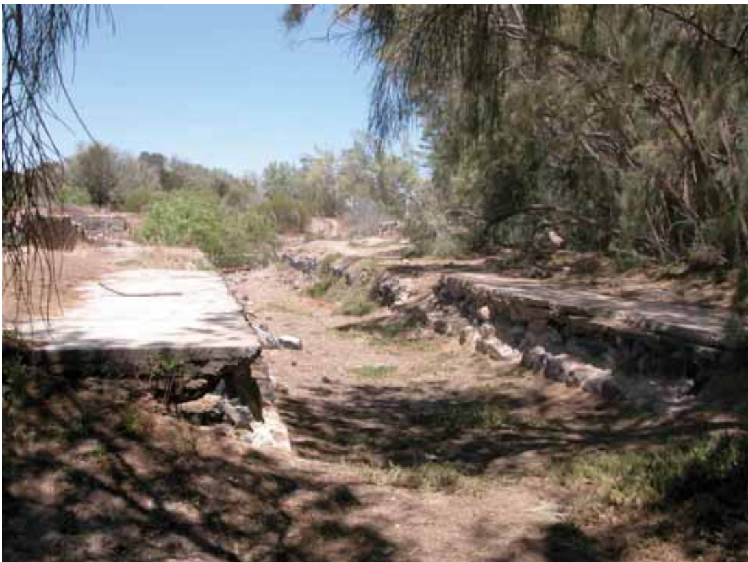
Fig 30 Some elements of the smelters such as the copper store stand outside the project area
