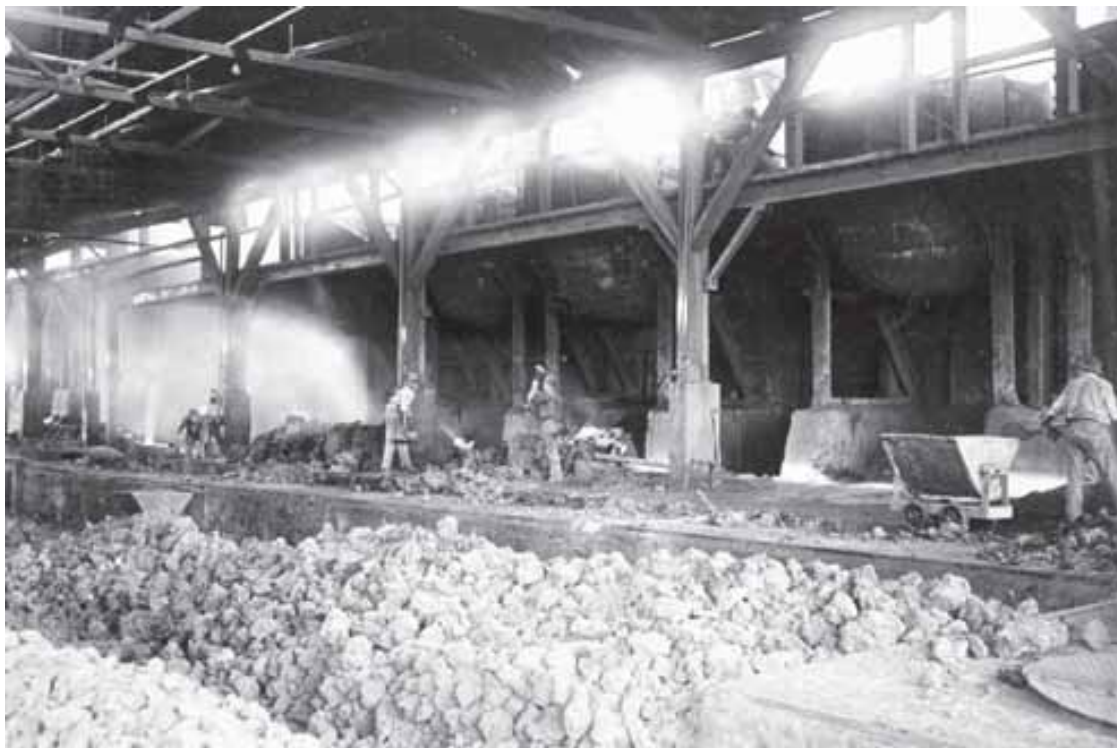
Fig 19 Breaking up the charge from the McMurtry sintering pots (PIRSA N020512a)
