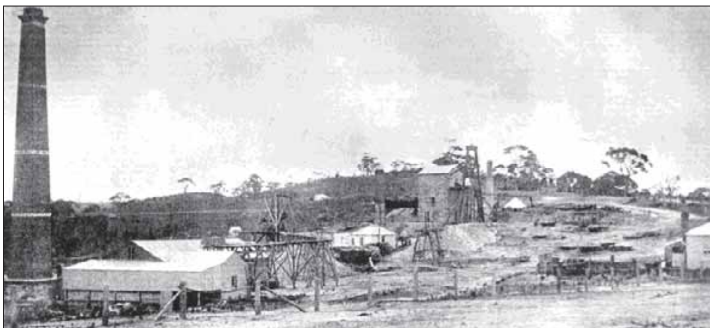
General view of the Bird-in-Hand Mine, 1899. At left is the battery house with an overhead tramway leading to Old Main Shaft. At centre is a Cornish enginehouse containing a 50-inch pumping from Burra at Victoria Shaft. PIRSA Photo 033767
