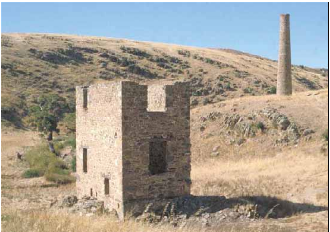
Worthing Mine Enginehouse, Hallett Cove
