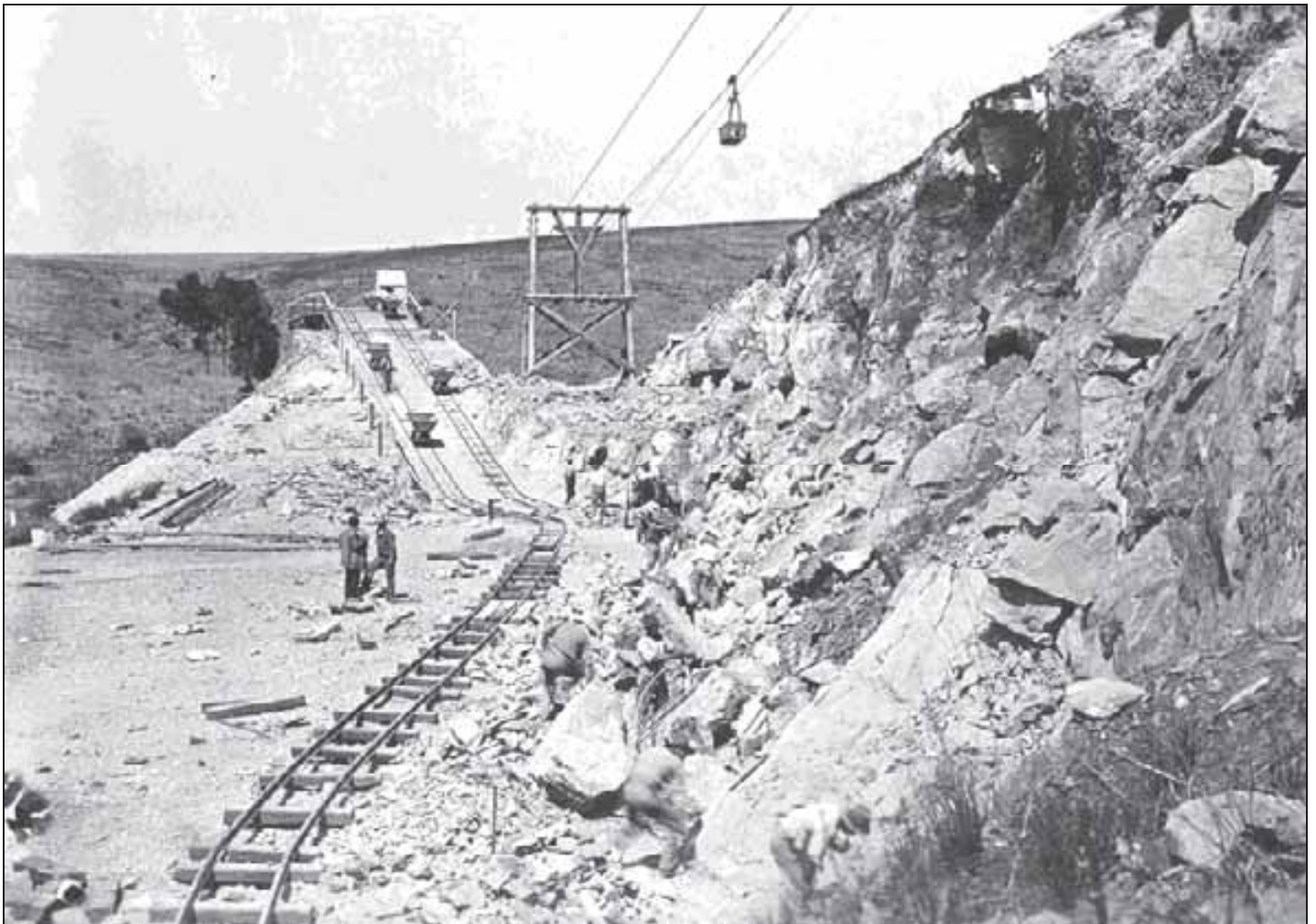
Old Reynella Quarry, 1928. Broken stone was hauled along the rail line to the crushing plant and aerial ropeway loading station in the background. PIRSA Photo N005070
