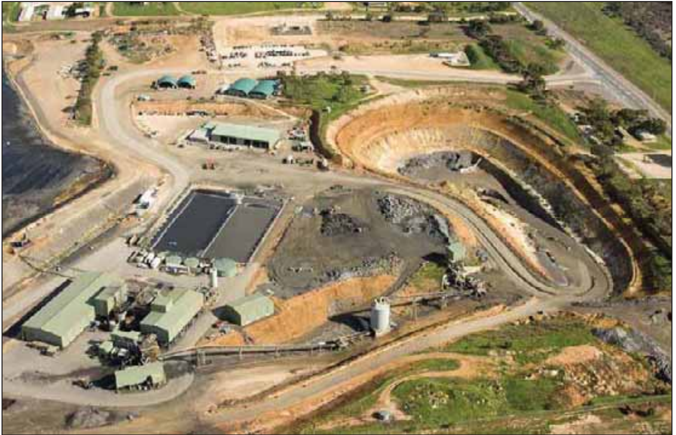
Aerial view of the Angas Mine open cut and treatment plant
