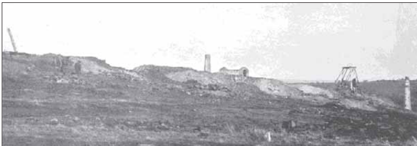
Wheal Ellen looking southeast, 1908. At the centre are the ruins of the pumping enginehouse and the tall chimney marks the site of the blast furnace. PIRSA Photo 034143
