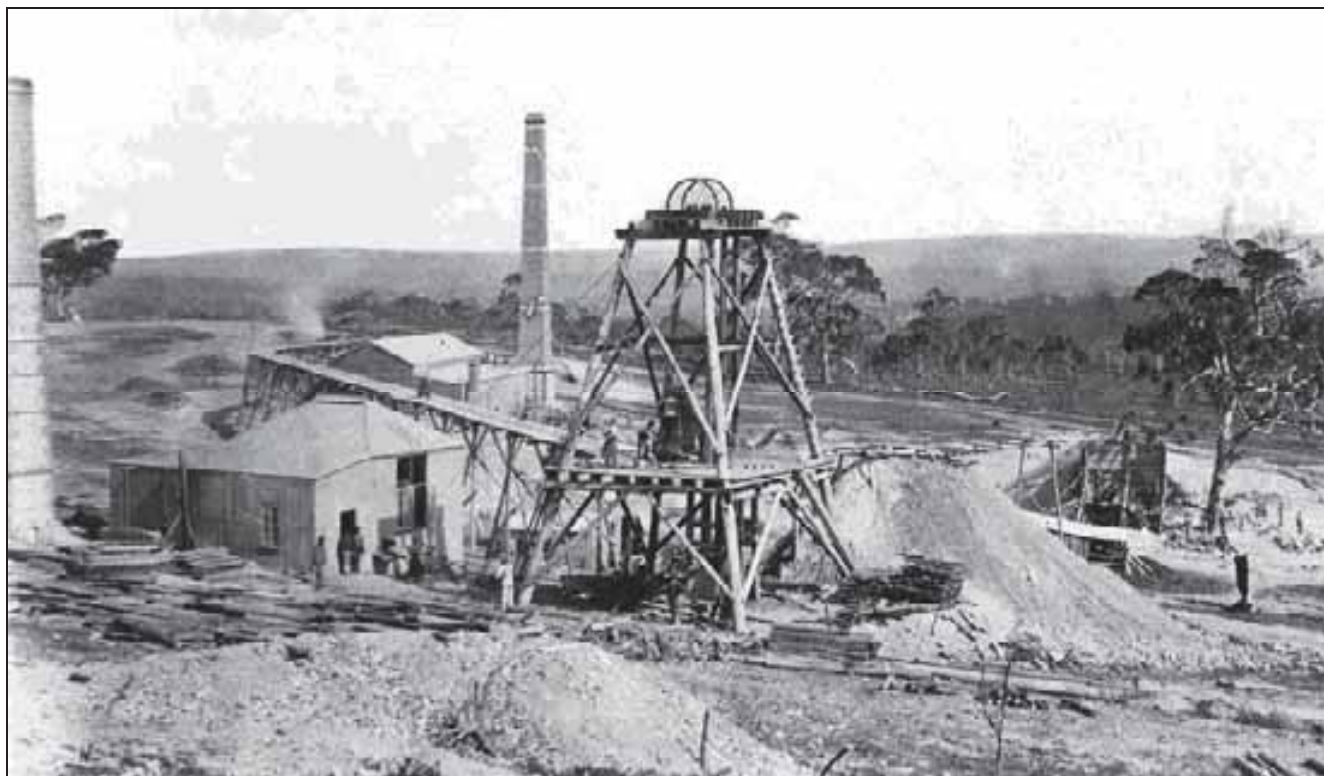
Bird-in-Hand Mine c.1883. At centre is Old Main Shaft and adjacent winding engine. The tramway takes ore to the battery in the background. PIRSA Photo 032948
