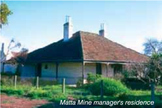
Matia Mine manager's residence
