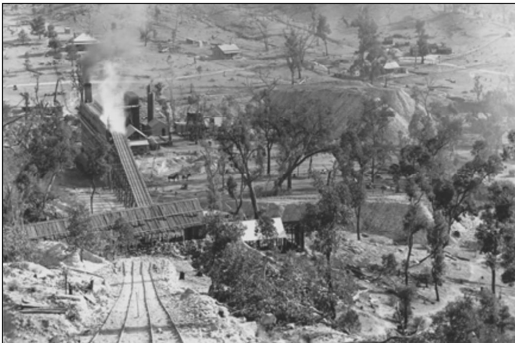
Looking down on the 1800s Torbane refinery in the Capertee Valley that is part of the area about to be mined by Centennial Coal. Courtesy of Leonie Knapman
