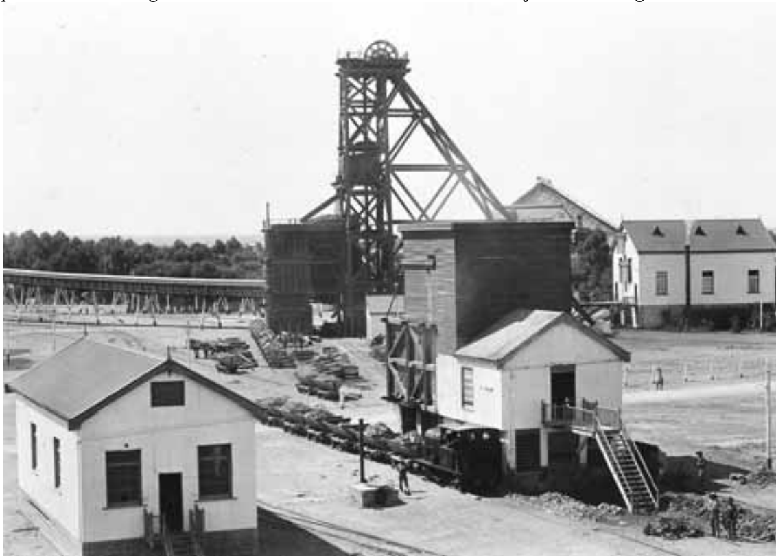
Attle Crushing Plant with Youngs Shaft in background, 1915
