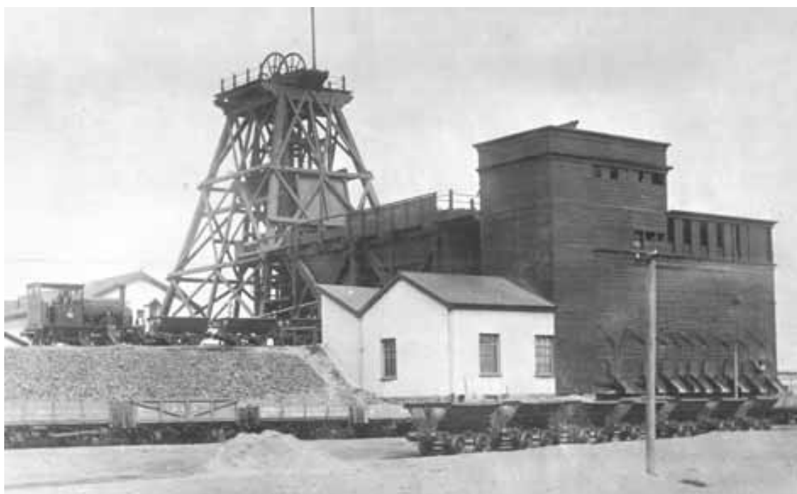
Taylors Shaft and sorting plant, c.1915
