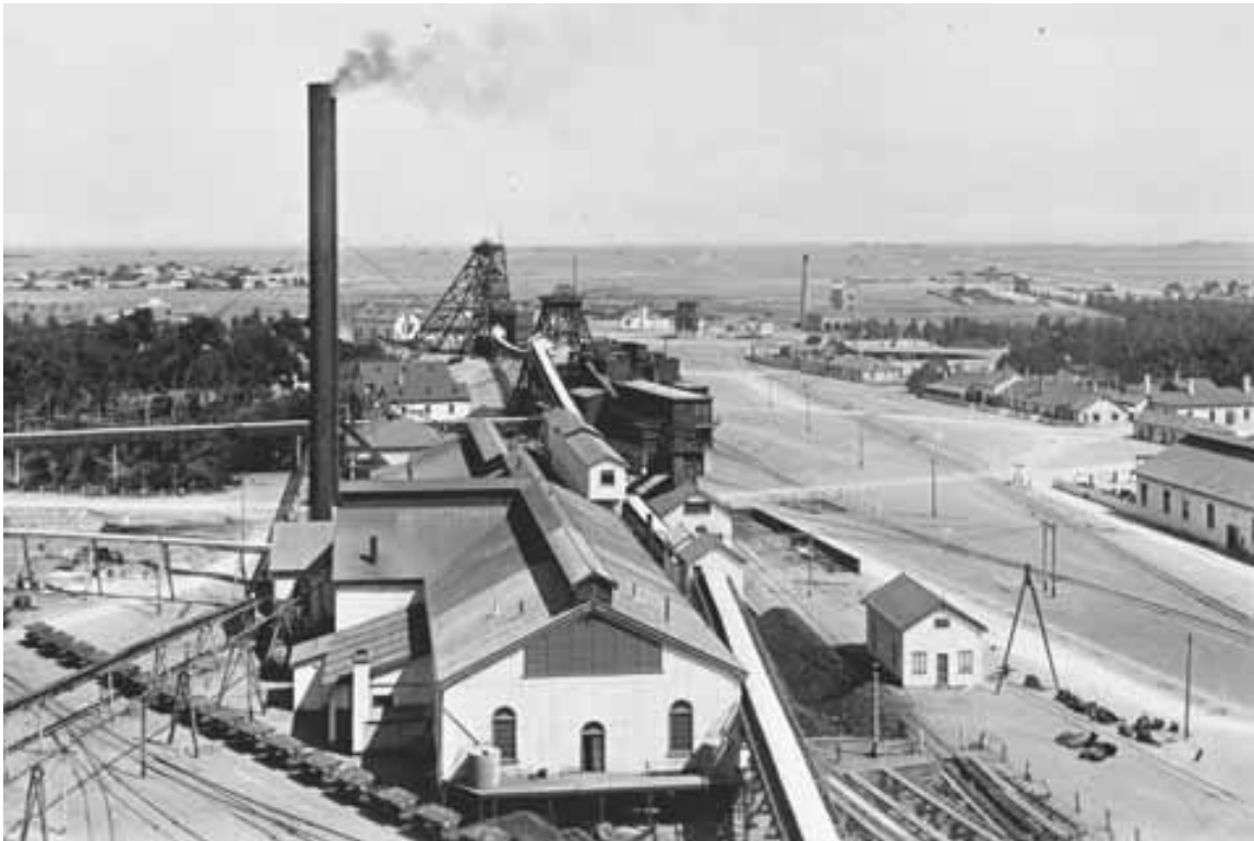
Wallaroo Mine looking west from Taylors Shaft, 1915. In the foreground is the powerhouse with Office sorting plant behind and Office and Youngs shafts
