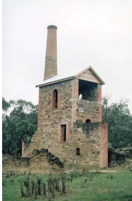
Engine house, Duke of Cornwall Mine , Fryerstown
