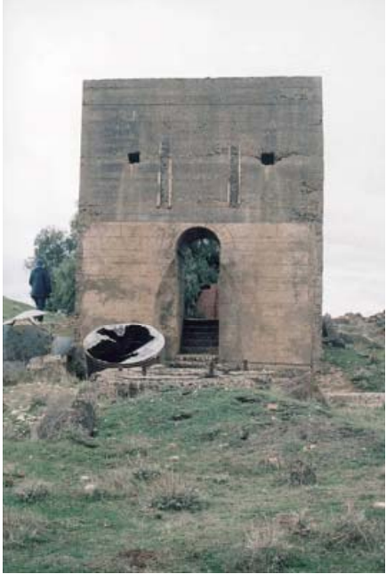
Cornish engine house, Victoria Gold Estates No.1 Shaft , near Smeaton
