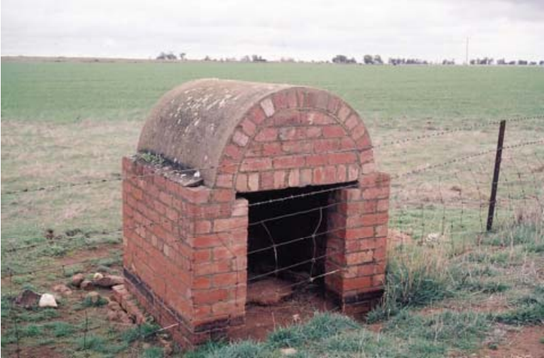
Brick magazine, Loddon Valley Goldfields Mine , near Carisbrook
