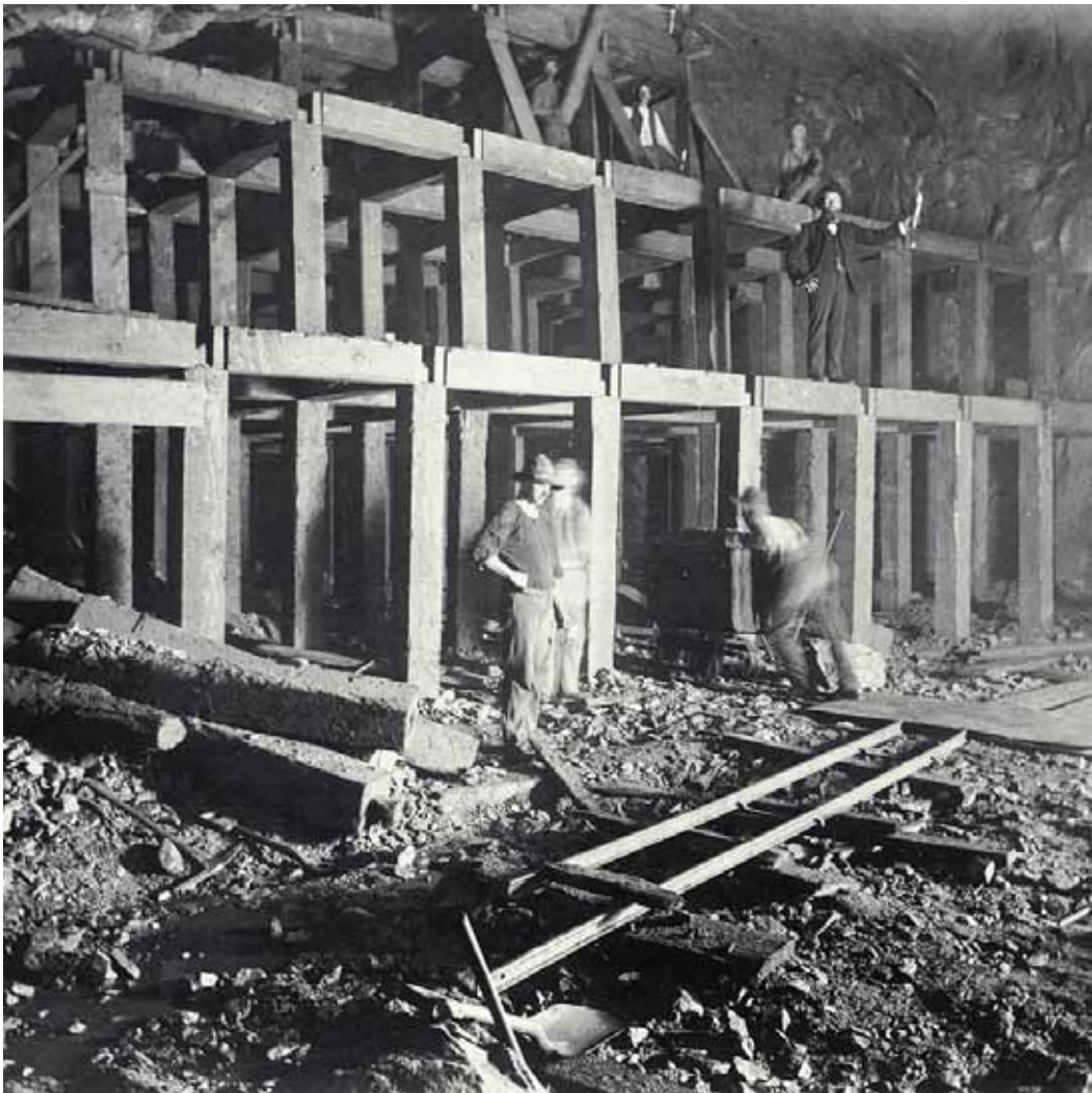
Set-square timbering, BHP Mine, Broken Hill, 1890.
