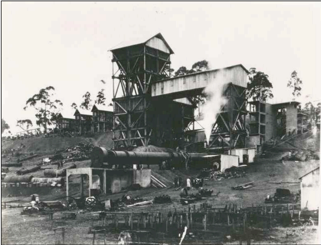
Figure 2: Shale works on the east bank of the Mersey River, circa 1924
