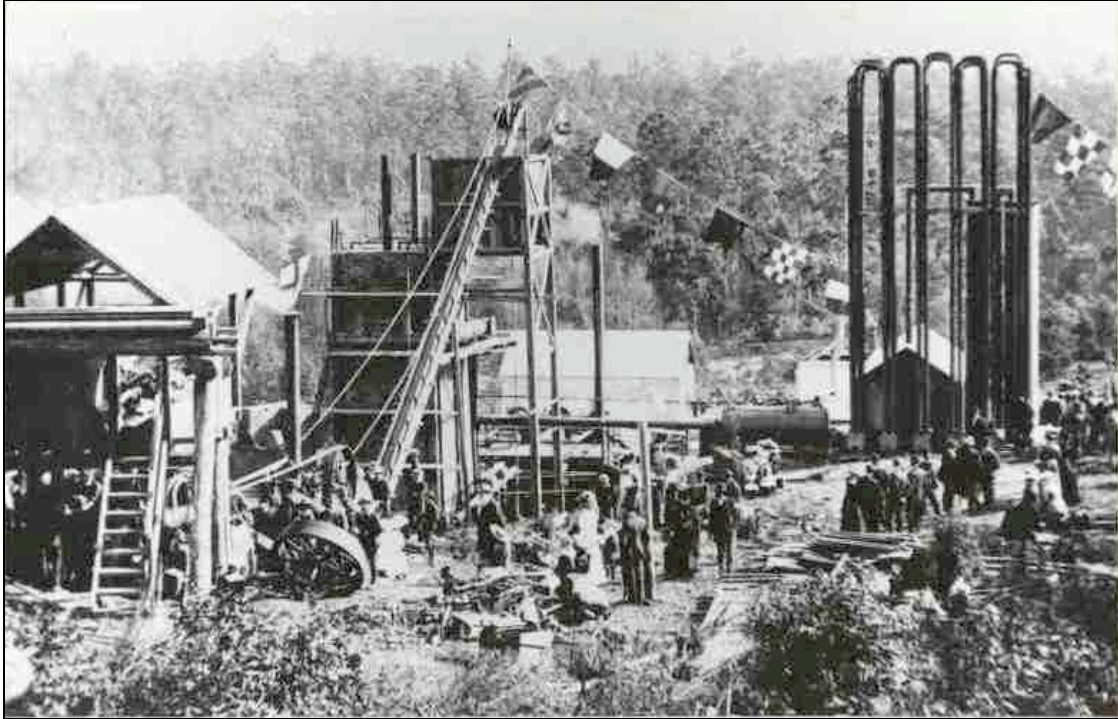
Figure 1: Shale works on the east bank of the Mersey River, circa 1912
