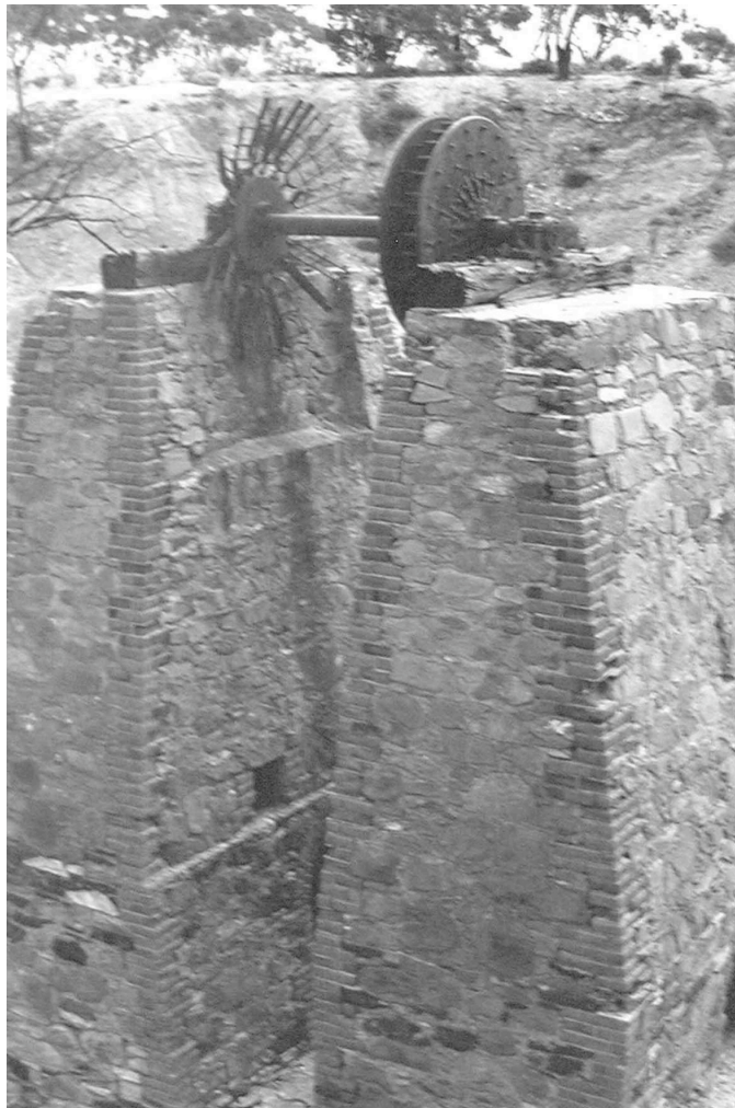
Photo 1: Tailings Wheel, Kings Battery.
